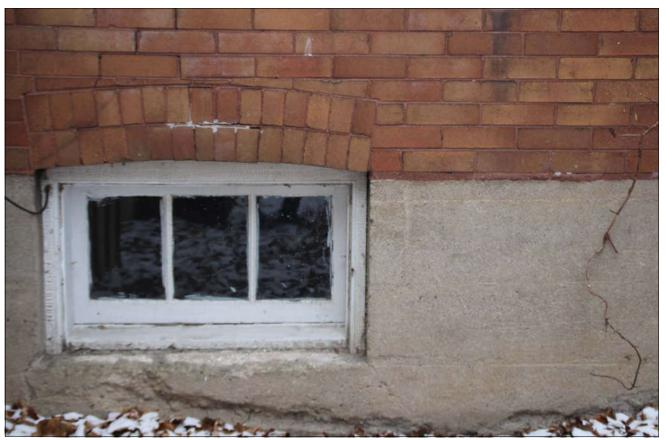
Figure 18 poured concrete foundation
