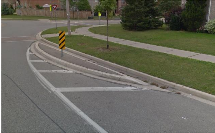
Figure 7 – Example Curb Extension at a Roundabout in Vaughan (Google)
