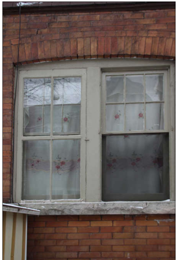
Figure 14 typical 6/1 paired windows (east side)
