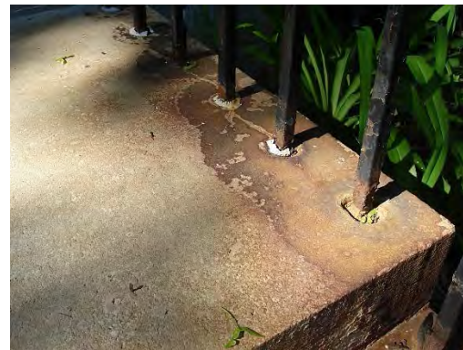
Advanced corrosion at base of metal pickets
