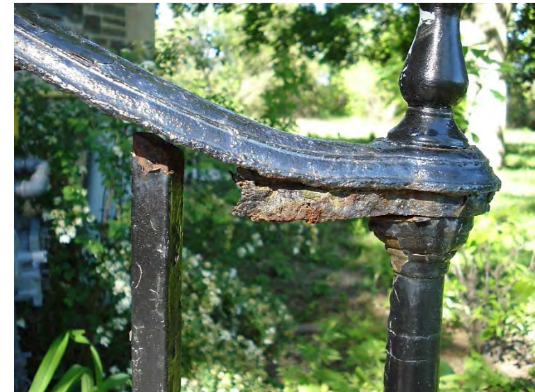
Loss of material due to corrosion at handrails
