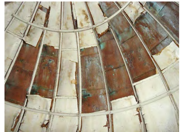
Deteriorated "Agasote" insulation
