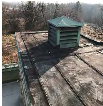
Old and deteriorated asphalt repairs over flat-seamed copper roofing.
