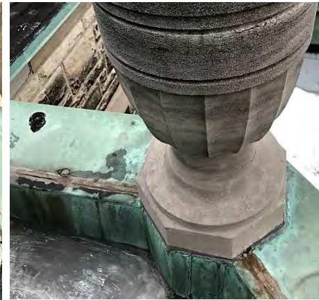
Deteriorated cap flashing and thru wall flashing
