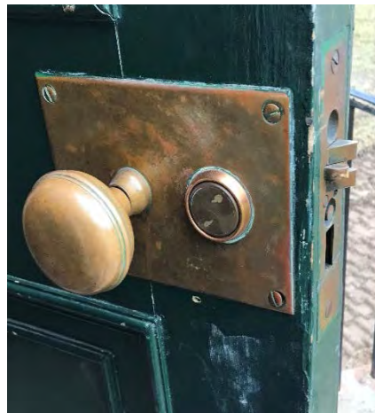
Heritage hardware requires cleaning and lubrication
