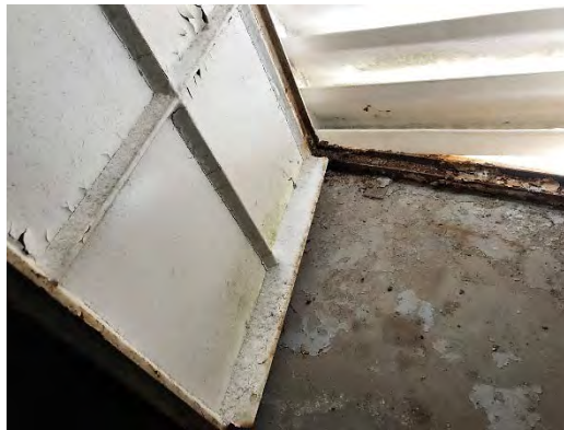
Rusting of windows and deterioration of putty
