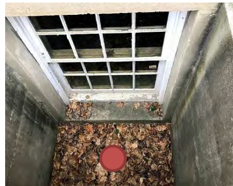
Poor & inefficient drainage in window wells
