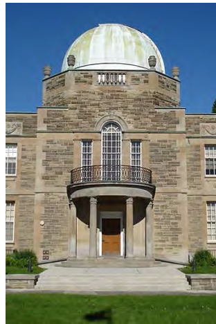
Main portico and entry steps with atmospheric soiling
