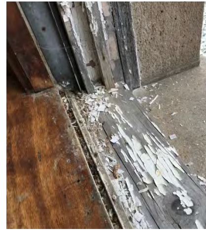
Extensive deterioration of finishes and weatherstripping at windows
