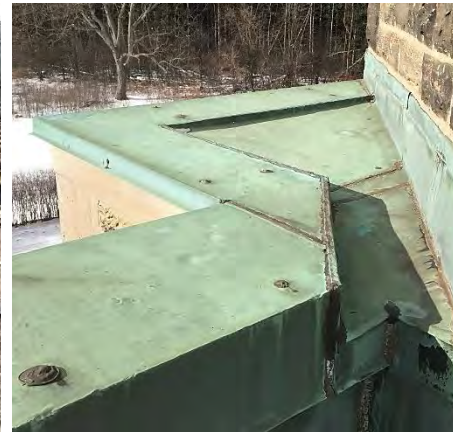
Old and deteriorated cap-flashing and joints between dif. materials
