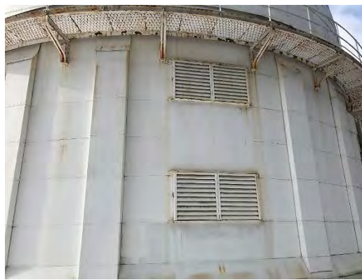
Corrosion and staining of exterior metal surfaces
