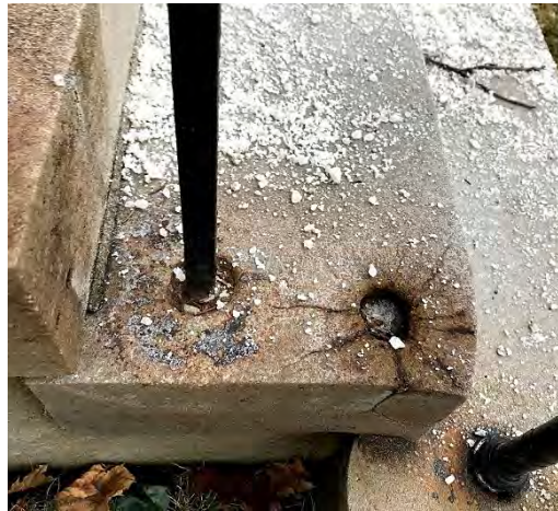
Cracks at stone threads of entry stairs and rust staining
