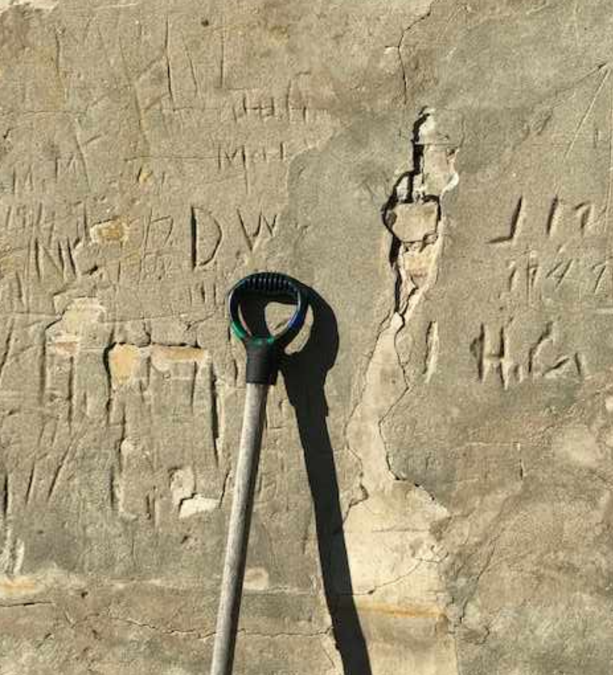
2j- Stucco, east elevation
