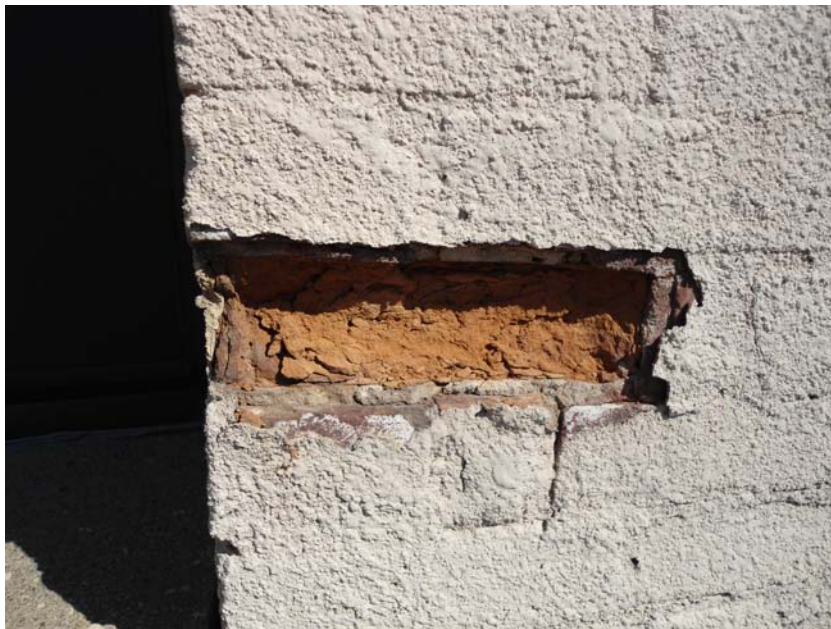
Figure 20: Spalled brick
