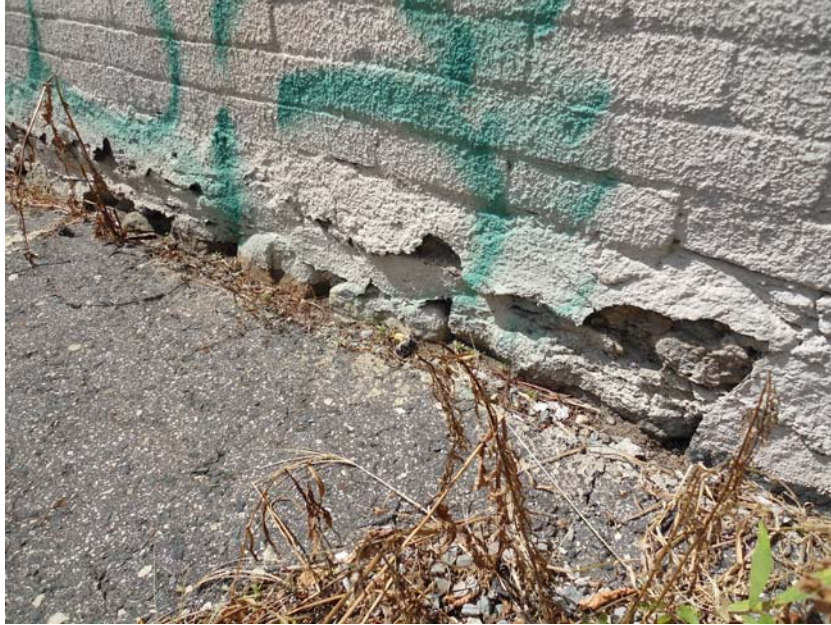
Figure 28: Exterior foundation at grade
