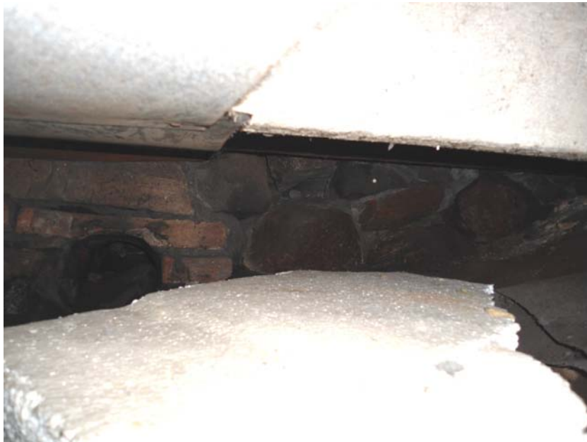
Figure 29: Exterior foundation wall at crawl space
