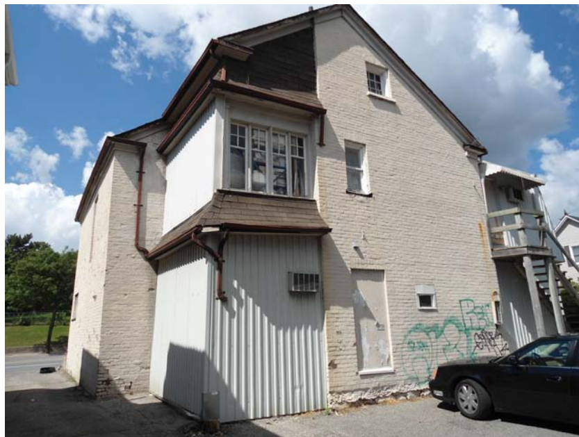
Figure 25: View of 2 storey sun room addition at southeast corner.
