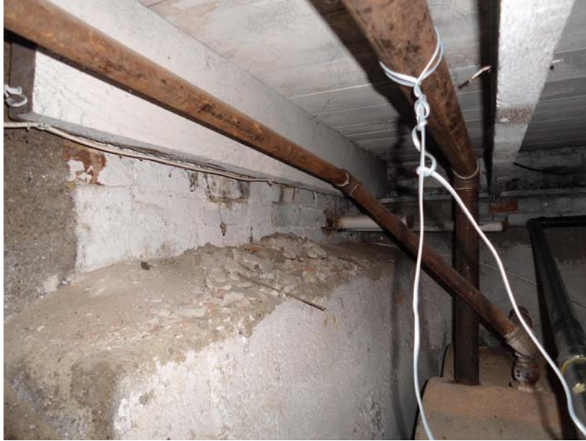
Figure 32: Poured concrete wall adjacent to north foundation wall
