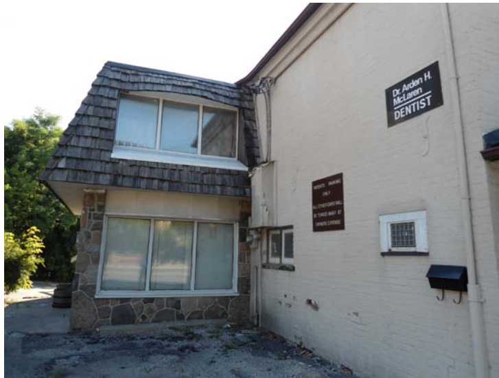
Figure 26: 2 storey 1960's addition view from Yonge Street
