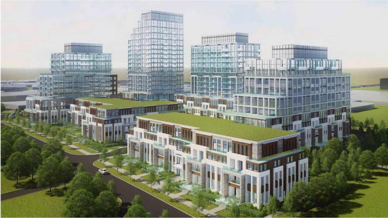
AERIAL VIEW LOOKING SOUTH WEST ALONG ARNOLD
