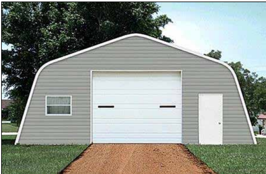
Figure 3: Example of the type of front façade the owner wishes to add to the metal structure (image provided by the owner).
