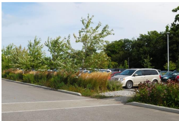
FIGURE 2.4-5 EDWARD GARDENS IN TORONTO PROVIDES BIOSWALES AND TREE PLANTINGS AS EXAMPLES OF LOW-IMPACT DEVELOPMENT IN A PARKING LOT.
