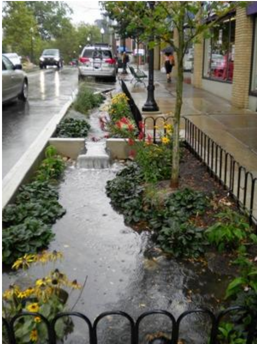
FIGURE 2.2-5, EXAMPLE OF LOW IMPACT DEVELOPMENT TECHNIQUE IN MILLBURY, MA
