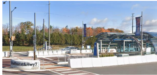
FIGURE 2.3-7 PRESENTLY THE BATHURST AND HIGHWAY 7 AREA PROVIDES A BRT STATION AT ENTRANCE TO RICHMOND HILL
