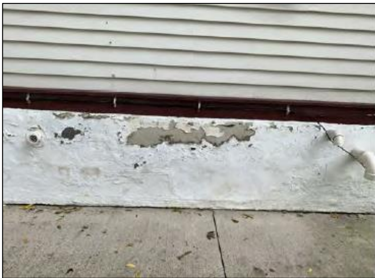
Figures 4 and 5: Example of foundation area and window sill that need repairing and repainting.
