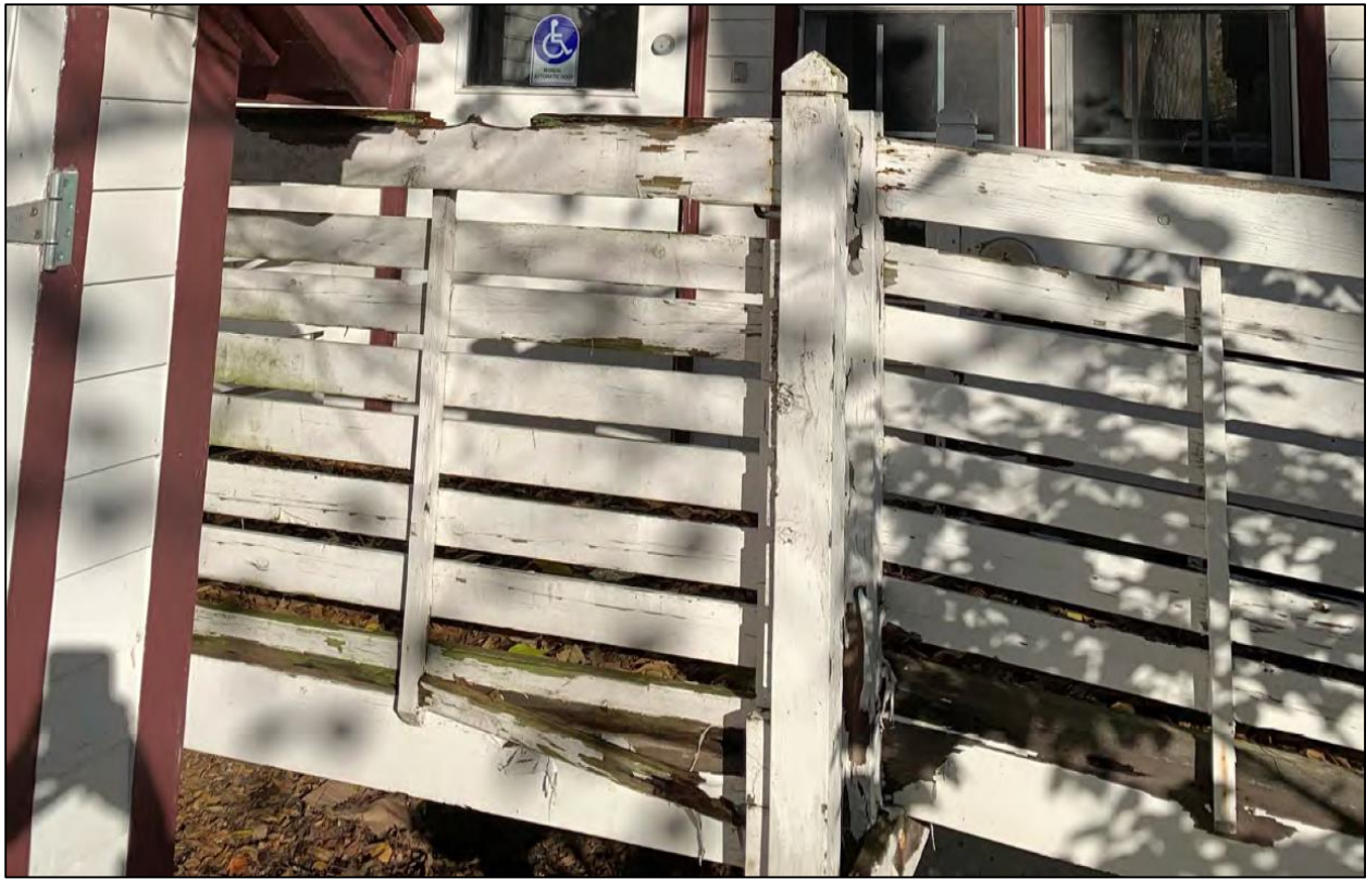
Figure 3: Example of wood rot in existing ramp.
