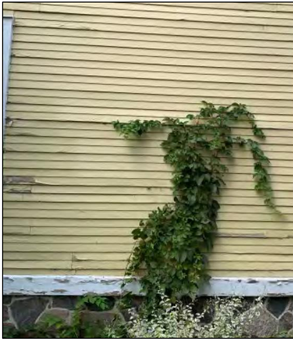
Figures 1 and 2: Photographs of the east elevation showing portions of the wooden siding and skirting board that require repairs and repainting, as well as climbing vines that are to be removed (left), and a door sill that requires repainting.
