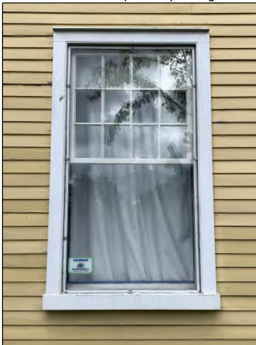
Figures 3 and 4: Photographs of a window with missing muntins (left), and of the basement door with a rusted frame (right).
