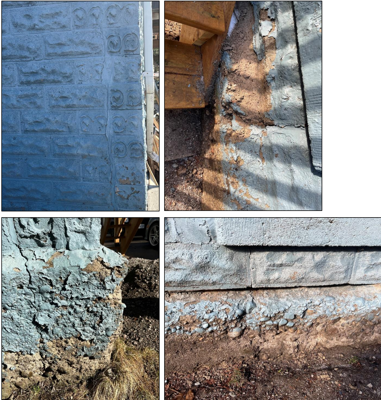
Figures 12 to 15 (clockwise from top left): Example of area that requires tuckpointing. Three photos illustrating areas of the foundation that require repair.
