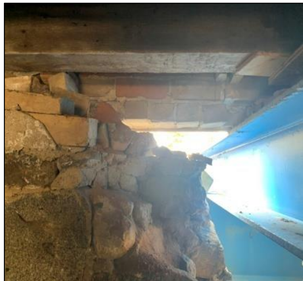
Figures 1 and 2: The existing condition of the David Hislop House on a structural platform (left) and an example of an exterior load-bearing wall not being properly supported (Soscia Engineering Ltd., 2021).
