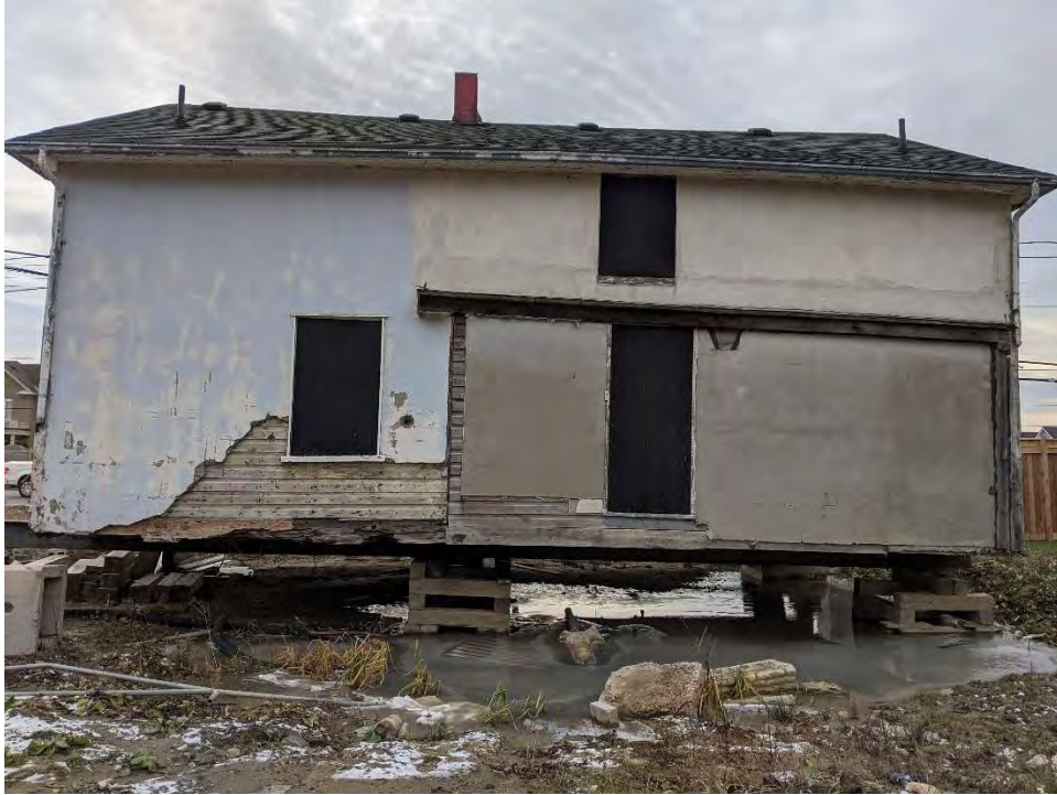
Photo 1. North elevation of John Love house.
