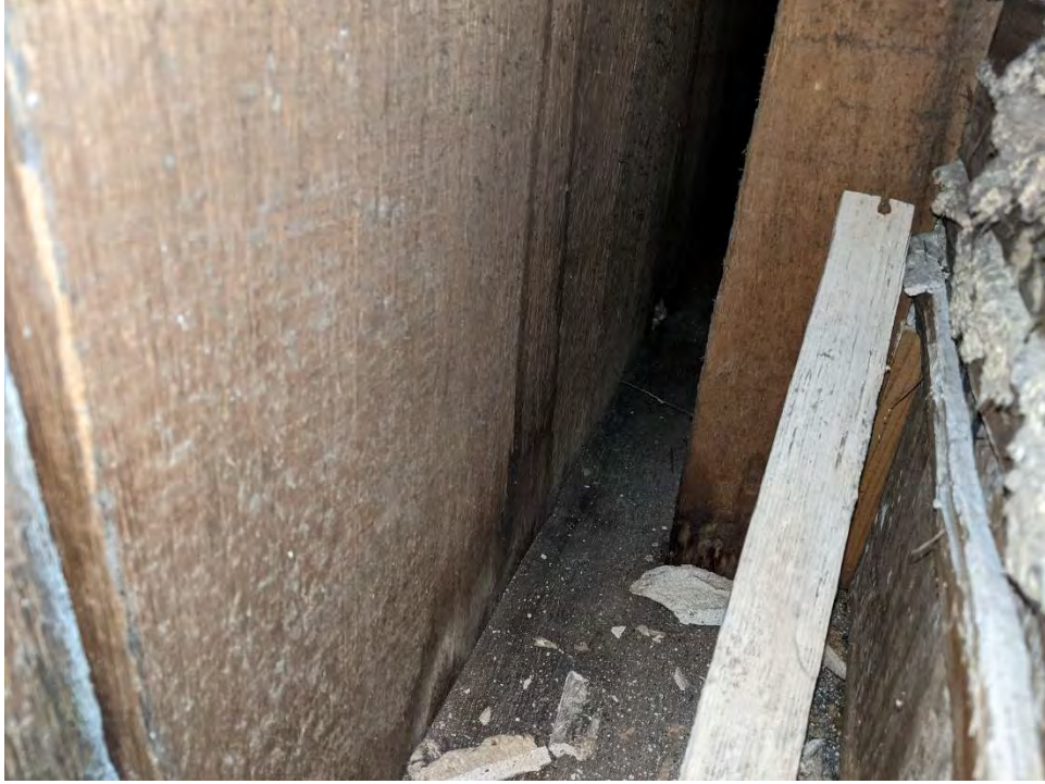
Photo 12. 2x4 stud wall in exterior wall of bedroom 4.
