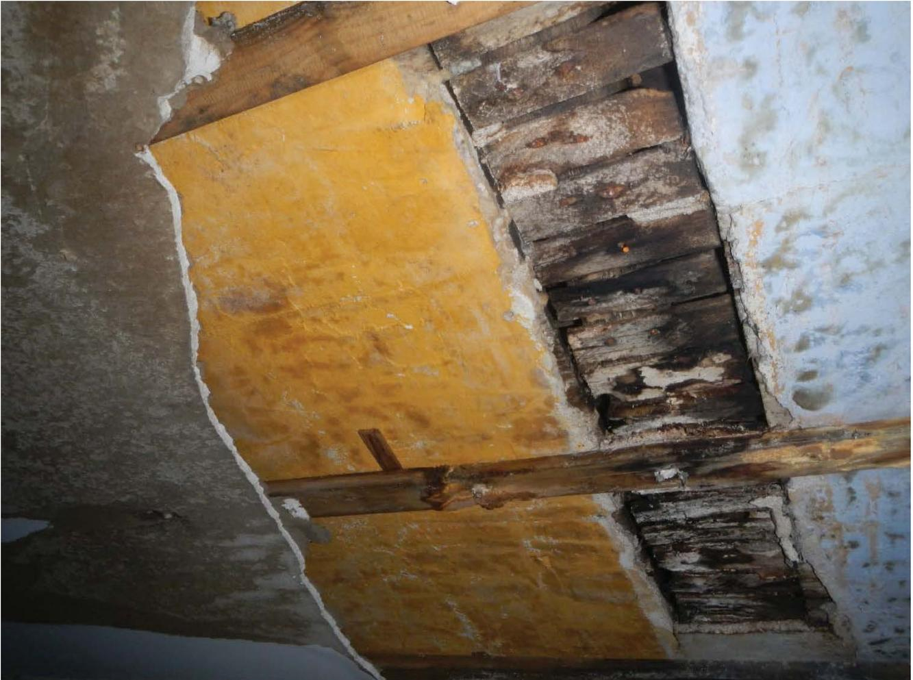
Ceiling of second floor showing water damage and mold
