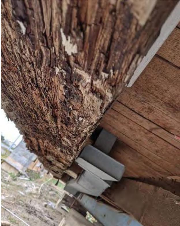
**Decayed south sill beam and failed adjacent floor joist.**
