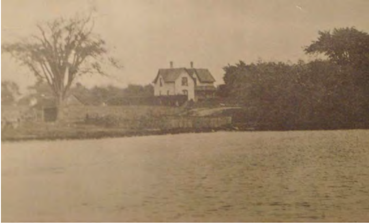
Undated photograph of the north and west elevation of the David Hislop House (c.1877), mill pond and dam associated with the Headford Mills (City of Richmond Hill).
