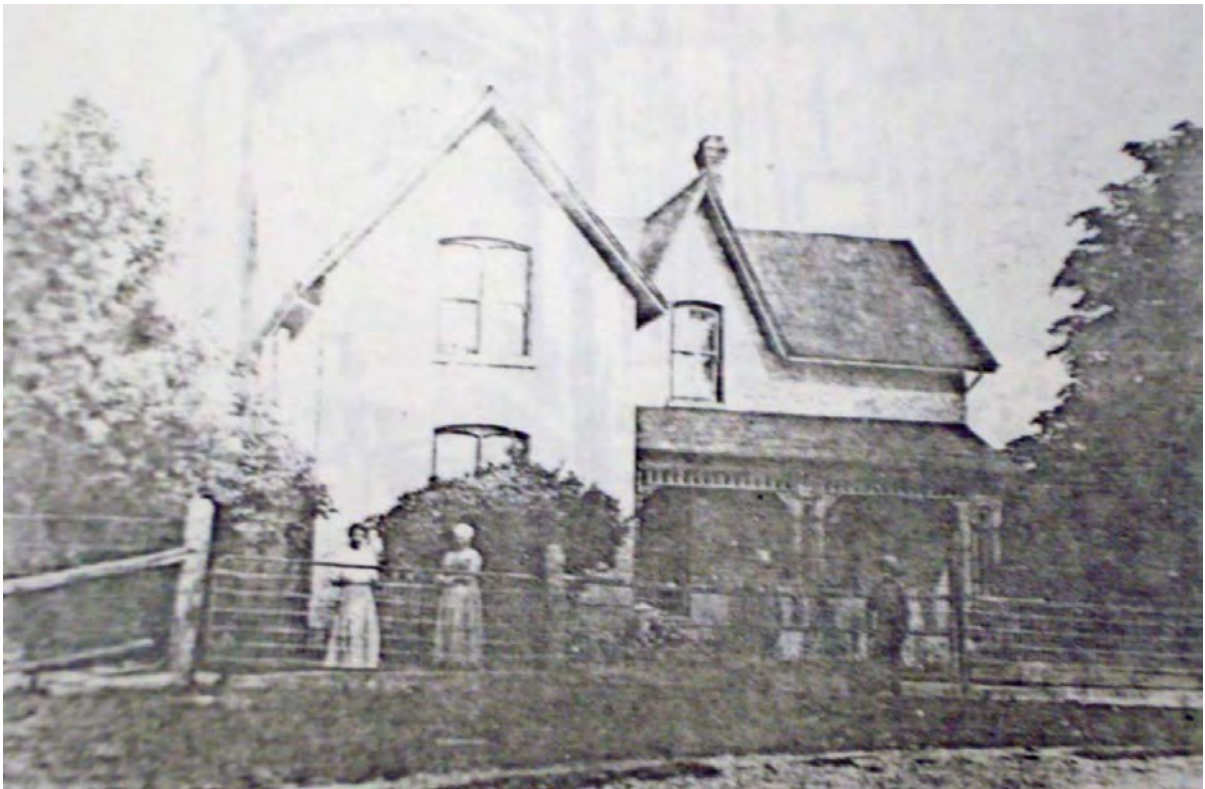
c. 1900 photograph of the west elevation of the David Hislop House, located directly adjacent to the Mill Complex (Champion).
