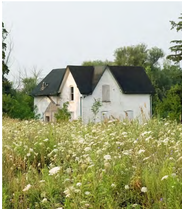
East and north elevation of the David Hislop House. A later addition to the east elevation has been removed (ERA, 2021).
