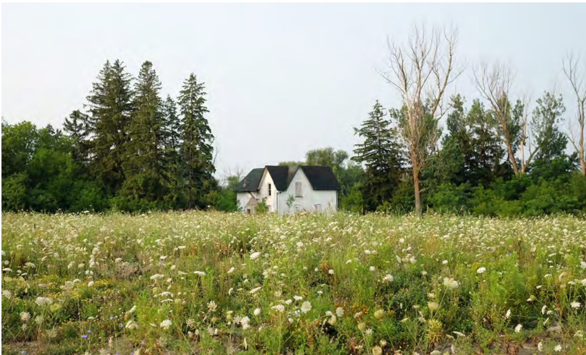
Looking towards the east and north elevation of the David Hislop House. The Site is unoccupied and the former Headford Mills and barn structures have since been demolished. The David Hislop House is currently sitting on a structural platform (ERA, 2021).
