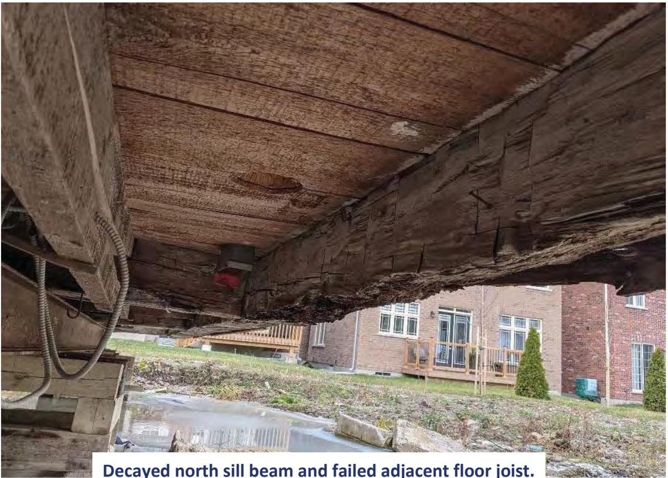
**Decayed north sill beam and failed adjacent floor joist.**
