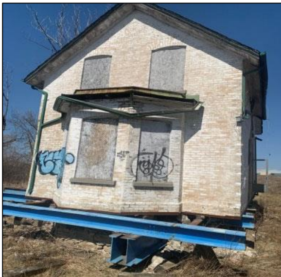
Figures 1 and 2: The existing condition of the David Hislop House on a structural platform (left) and an example of an exterior load-bearing wall not being properly supported (Soscia Engineering Ltd., 2021).
