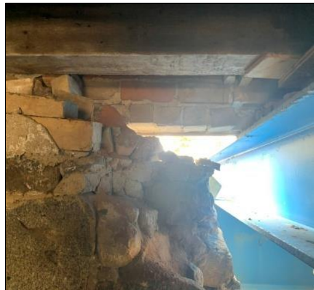
Figures 1 and 2: The existing condition of the David Hislop House on a structural platform (left) and an example of an exterior load-bearing wall not being properly supported (Soscia Engineering Ltd., 2021).
