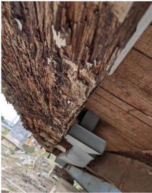
Decayed south sill beam and failed adjacent floor joist.
