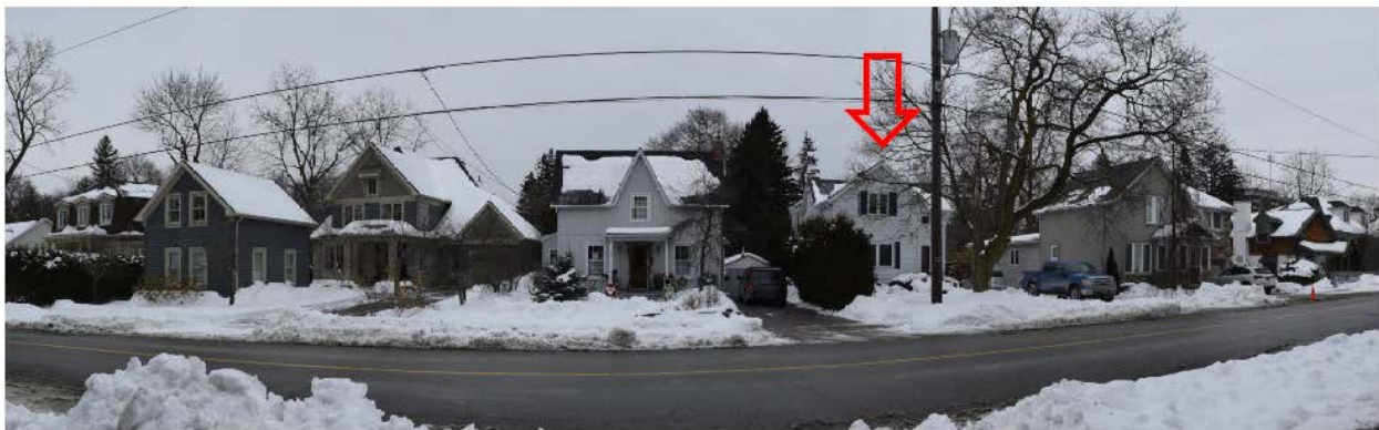
Figure 2: Composite image of street scape, with red arrow indicating location of 83 Arnold Crescent (PHC Inc.).
