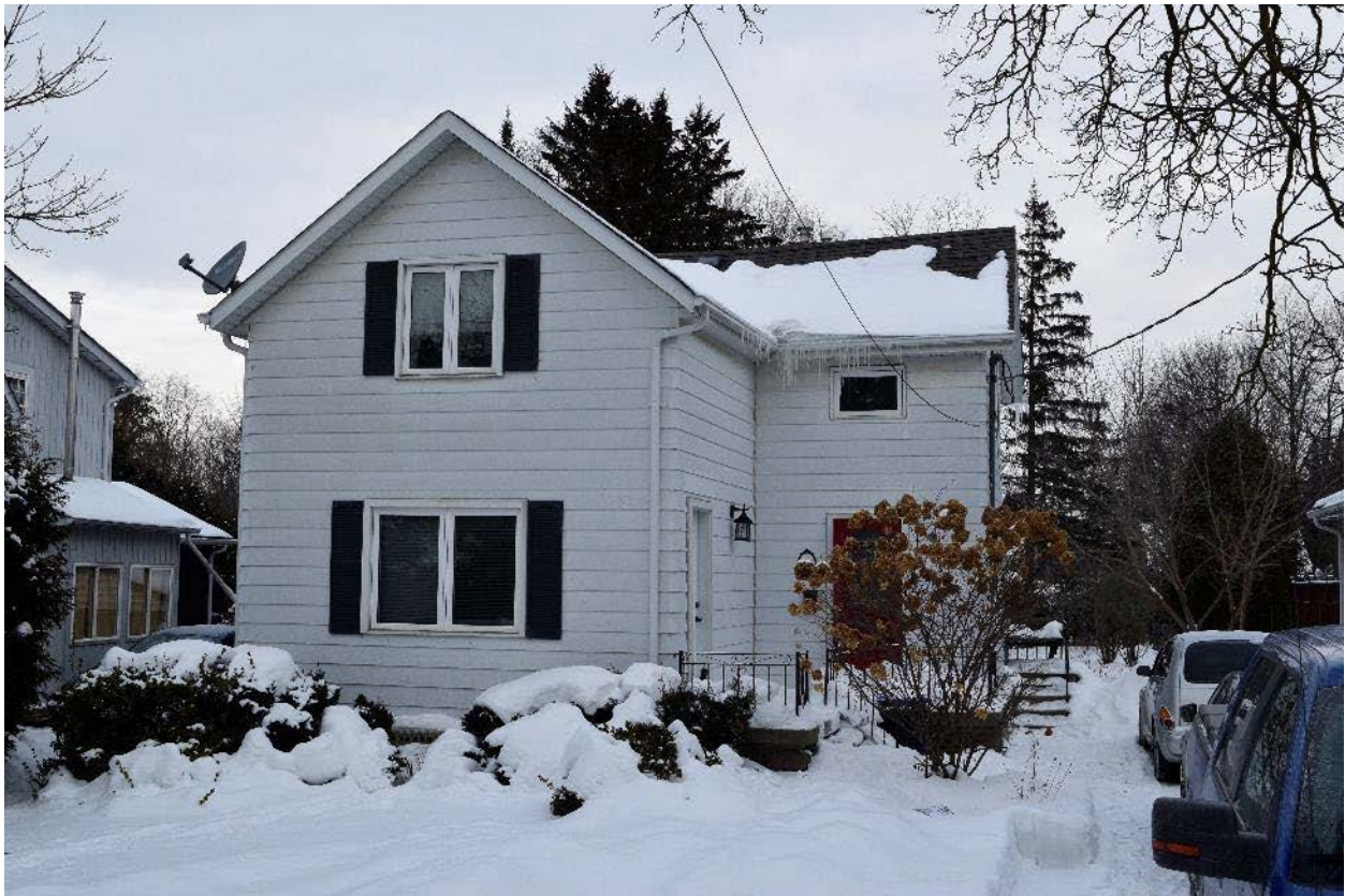
Figure 1: The subject property as viewed from Arnold Crescent (PHC Inc.).
