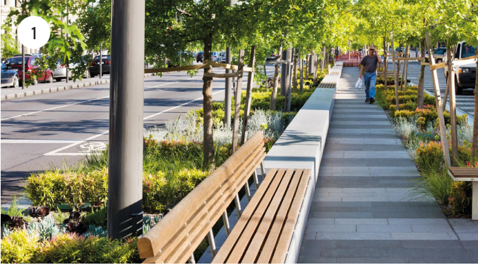
Pedestrian Connection - Lonsdale St, Dandenong, Australia
