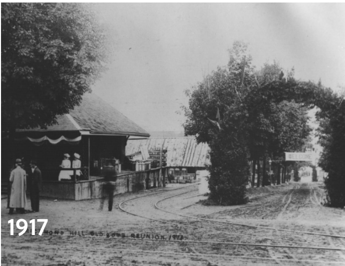
FIGURE B-5 Lorne Street Looking East to Town Park
