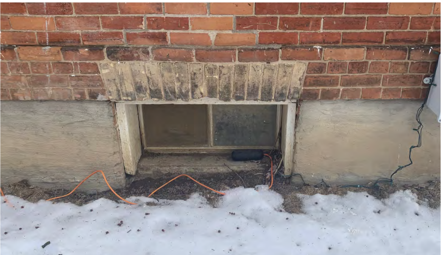
View of Basement Window West Elevation
