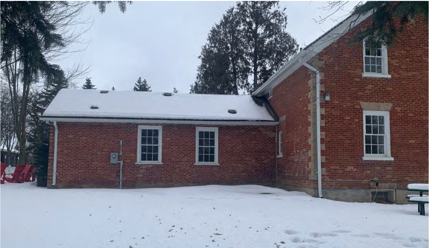
West Elevation at North
