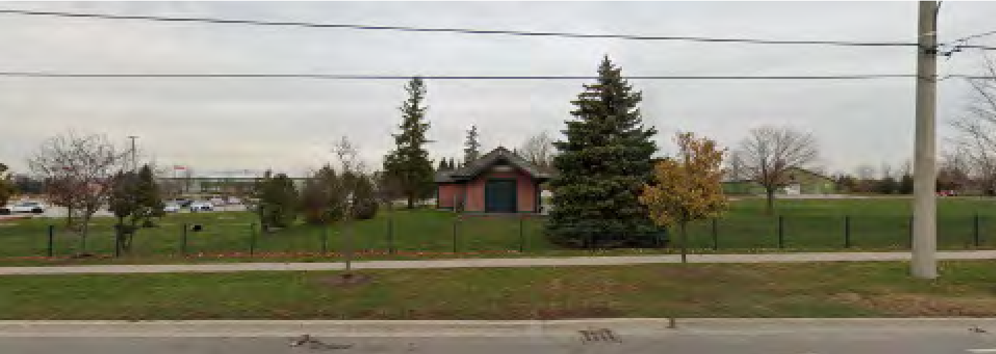
Streetscape North of Elgin Mills Road East - Subject Property at 1370 Elgin Mills Rd E
