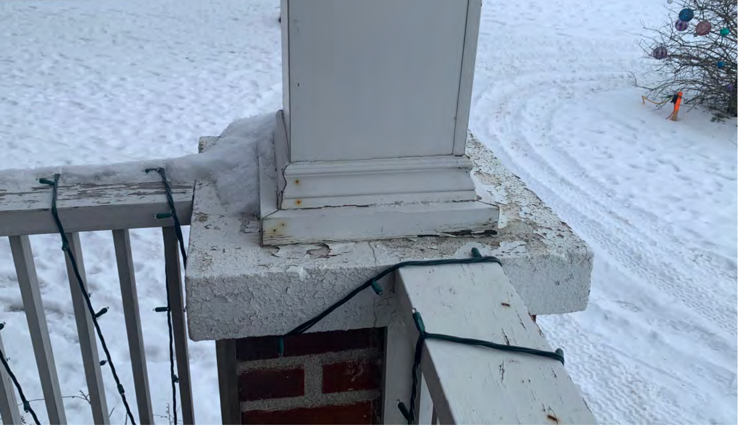
View of Base of East Porch Column
