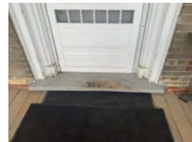
PHOTO 1.1 - REPAINT DOOR THRESHOLD AND FRAME
