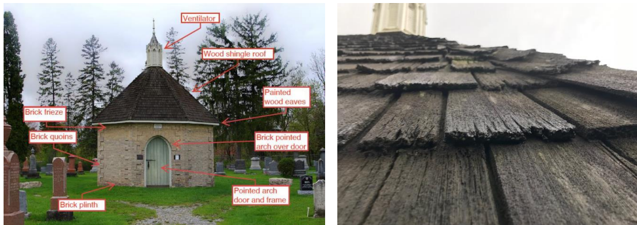
Figure 2 Image showing the Octagonal Vault's architectural elements (left), and a detailed view of the building's existing highly deteriorated wood shingles (right), which are proposed to be replaced with a new asphalt roof.
