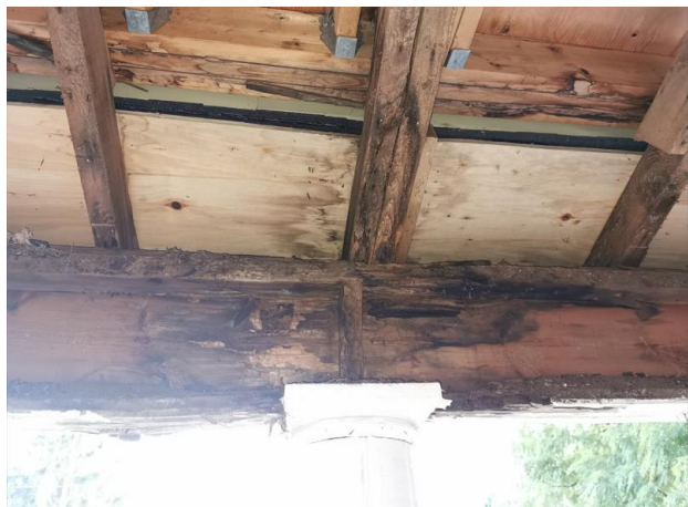
Figure 1 Photographs showing the extent of water damage to the structural elements of the front verandah/balcony at 188 Gormley Rd. W. in 2019 (left) and 2022 (right).
