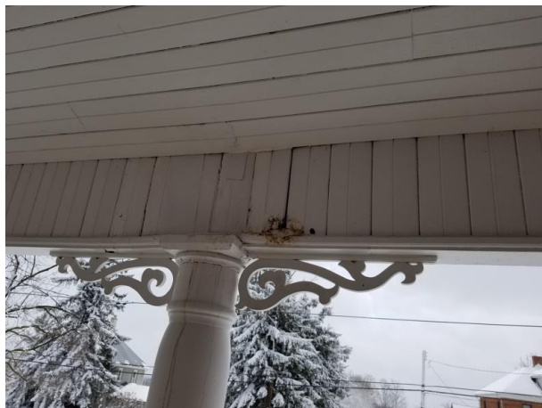
Figure 1 Photographs showing the extent of water damage to the structural elements of the front verandah/balcony at 188 Gormley Rd. W. in 2019 (left) and 2022 (right).
