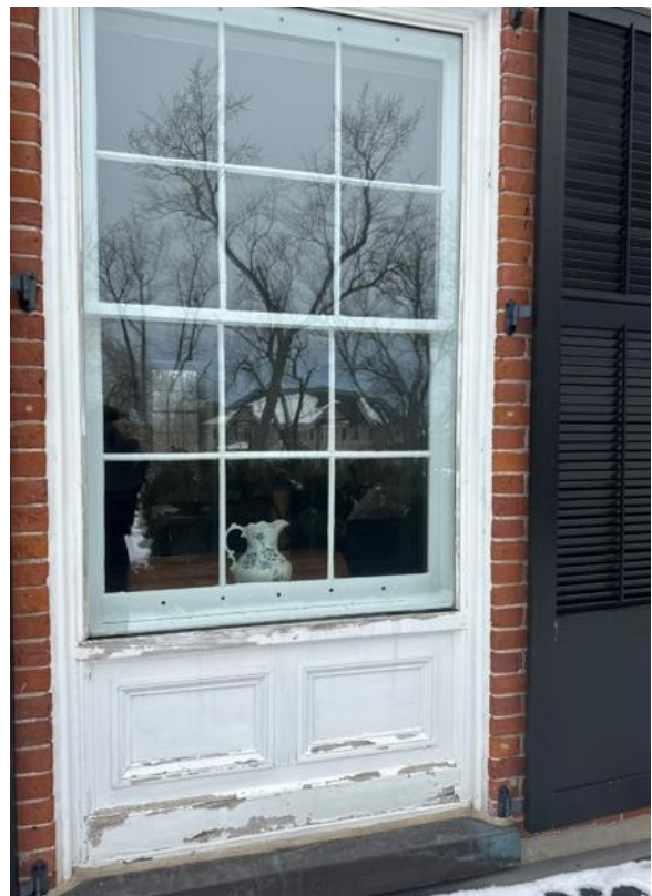
Figure 6 Photographs showing 16 Macleod Estate Ct.'s front (south) entryway (left) and a typical ground-floor window, which are proposed to be repaired and repainted.
