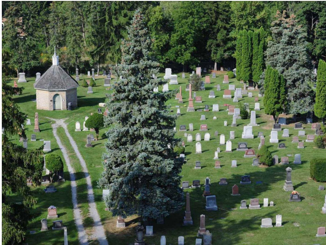
Figure 1 View of the Octagonal Vault within the Richmond Hill Presbyterian Church Cemetery (source: Edwin Rowse Architecture Inc.).
