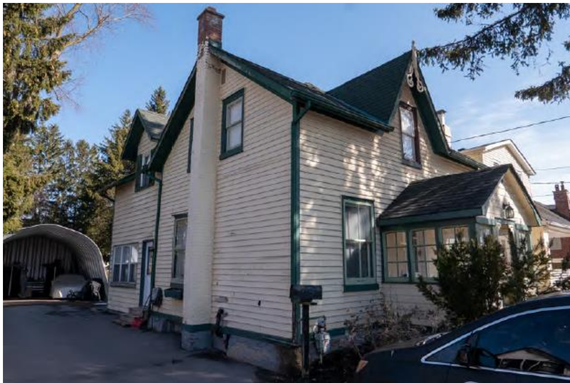
Figure 1 View northeast of the dwelling at 103 Richmond Street, showing the main (south) portion with non-original enclosed front porch in the foreground, rear (north) extension/addition in the background, and temporary steel garage structure on the far left (Source: CBCollective)
