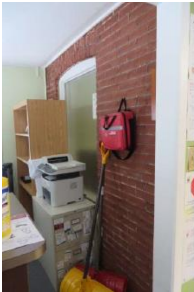
Figure 2 View of 9893 Leslie Street's original red brick cladding, visible from the interior of the enclosed front porch; note that this brick is now completely obscured by the irreversible application of a cementitious coating on the exterior of the building (Source: Stevens Burgess Architects Ltd.)
