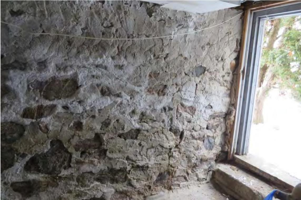
*Fieldstone Foundation (interior) with Significant Efflorescence*
