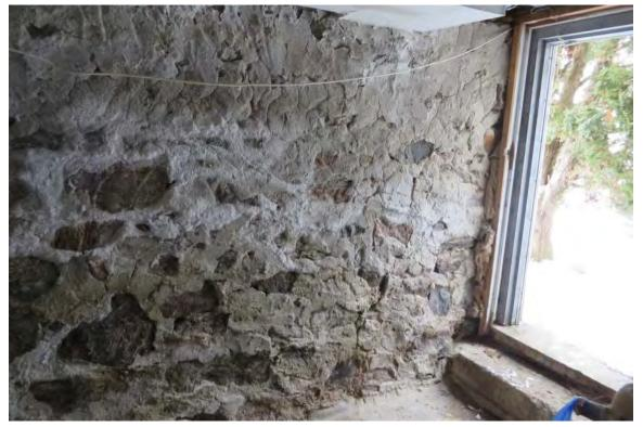
Fieldstone Foundation (interior) with Significant Efflorescence
