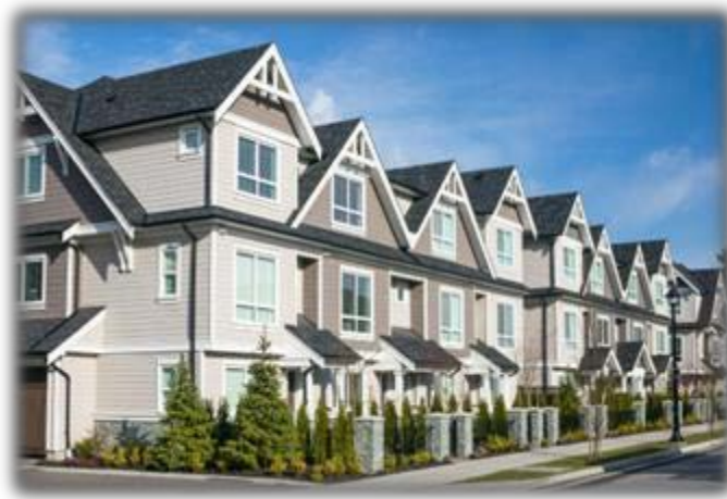
Figure 3-3 City of Richmond Hill Example of Townhouse
