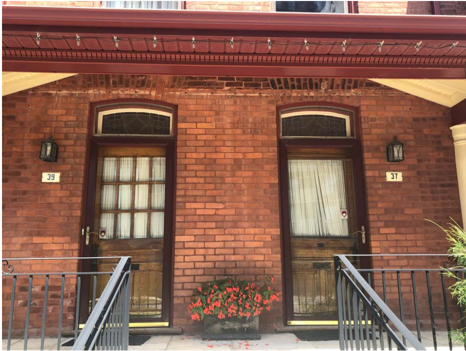
Figure 7 Detailed photograph of the front doors of 37 (right) and 39 (left) Centre St W, showing the original wood paneled doors with glazed upper sections and coloured art-glass transoms (Source: HUD, 2023).
