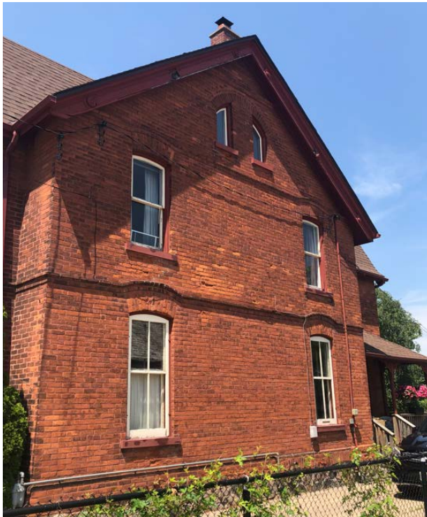
Figure 8 Photograph showing the side (east) elevation of 37 Centre Street West. Note the medium-pitched gabled roof with bargeboard trim, segmental-arched windows, slanting segmental-arched attic windows, brick stringcourses, and the original hip-roofed verandah at the rear (far right) with turned wooden posts and fretwork brackets with a stylized tulip motif (Source: HUD, 2023).
