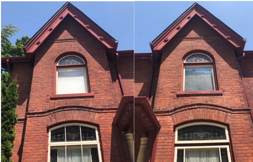
Figure 6 Detailed photographs of 37 (right) and 39 (left) Centre St W's projecting front bays, showing the coloured art-glass window transoms and sidelights, brick stringcourses and 'basket-weave' banding, and paneled bargeboards with bullseye motifs (Source: HUD, 2023).
