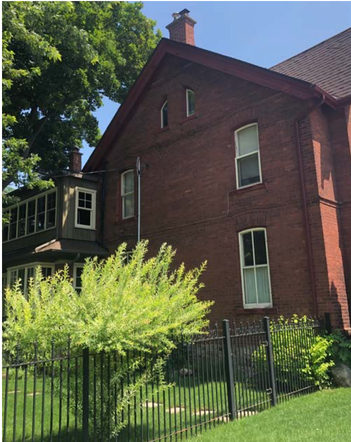
Figure 9 Photograph showing the side (west) elevation of 39 Centre Street West. Note the medium-pitched gabled roof with bargeboard trim, segmental-arched windows, slanting segmental-arched attic windows, and brick stringcourses. Also note the non-original rear sunroom addition on the far left (Source: HUD, 2023).
