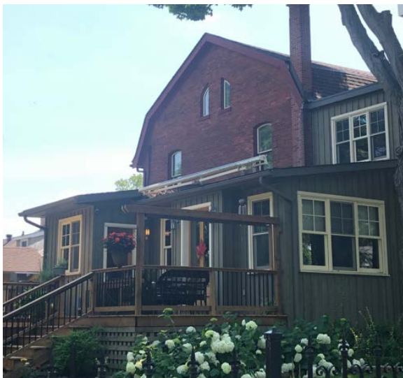
Figure 10 Photograph showing the rear (north) elevation of 37 and 39 Centre Street West. Note the gambrel roof and slanting segmental-arched attic windows (Source: HUD, 2023).
