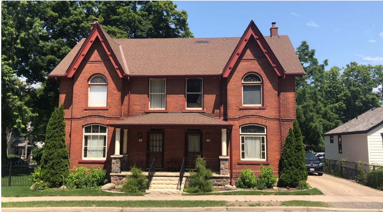
Figure 5 Photograph looking north, showing the front (south) elevation of the William Proctor Double House at 37 and 39 Centre Street West. Note the projecting front bays with steeply-pitched gables and segmental and round-arched windows with coloured art-glass transoms and sidelights, the red brick cladding with stringcourses and basket-weave patterns, and the asymmetrical design of each semi-detached unit (Source: HUD, 2023).
