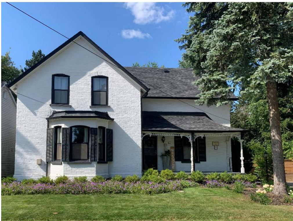
Figure 4 Current photograph looking north, showing the principal (south) elevation of 111 Richmond Street. Note the building's 1 ½ - storey massing, medium-pitched cross-gabled roof, bellcast-roofed verandah with turned wooden posts and decorative spindlework trim, and mansard-roofed bay window. (Source HUD, 2023).
