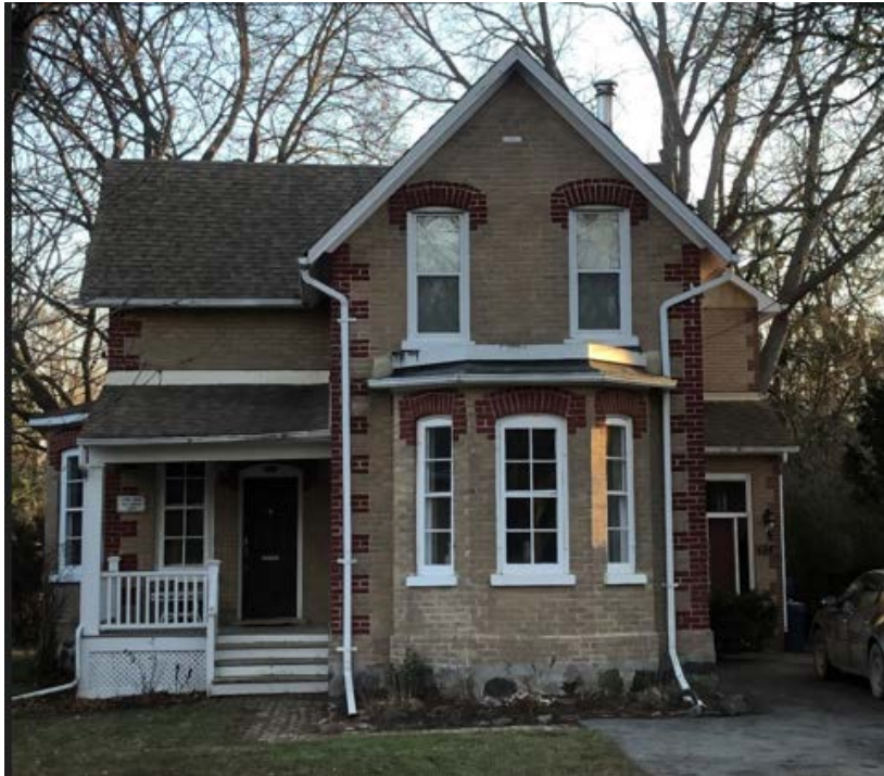
Figure 4 Photograph of 124 Richmond Street's front (north) elevation, looking south from Richmond Street. Note the building's 1 ½-storey massing, L-shaped plan, steeply-pitched cross-gabled roof, dichromatic brickwork with red-brick quoining and voussoirs/hood molds, projecting bay windows, and the 1888 date stone within the front gable (Source: HUD, 2023).
