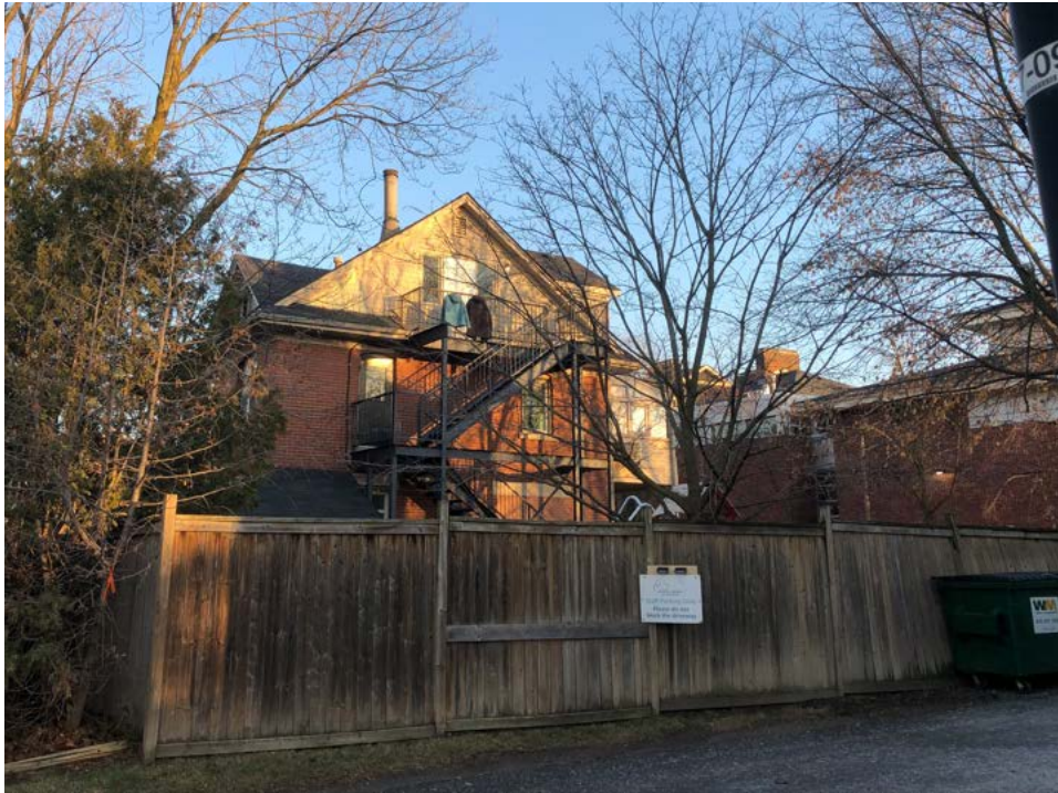
Figure 7 Photograph of the William Pugsley House's side (west), looking southeast from Arnold Crescent. Note that many window openings on this elevation have been altered to accommodate a fire escape (Source: HUD, 2023).
