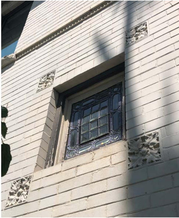
Figure 9 Detailed photograph showing the square, leaded art-glass window on the Andrew Newton House's south elevation, with corners punctuated by terra cotta tiles depicting stylized maple leaves. (Source: HUD, 2023).
