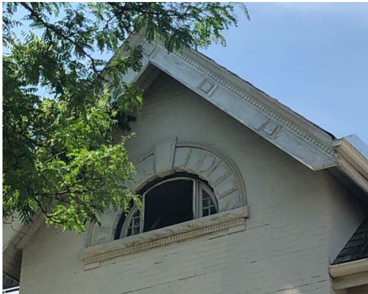
Figure 8 Detailed photograph showing the front (east) gable of the Andrew Newton House, with paneled bargeboards topped by dentiled trim, and half-round attic window opening on the principal (east) elevation, with a rock-faced lugsill, voussoir and keystone, surrounded by angular-cut masonry detailing, and containing a period wood unit divided in three sections, with multi-paned sidelights. (Source: HUD, 2023).
