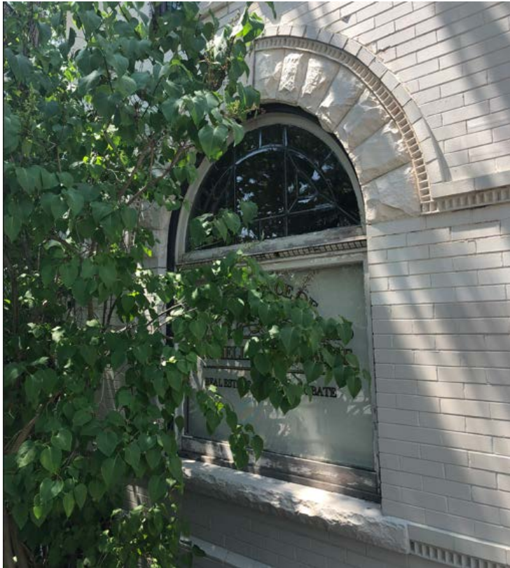
Figure 7 Detailed photograph showing the round-arched window opening at ground-floor level of the Andrew Newton House's principal (east) elevation, with a rock-faced lugsill, voussoir and keystone, topped by masonry stringcourse detailing, and containing a period wood window unit, with a leaded art-glass transom and dentiled trim. (Source: HUD, 2023).
