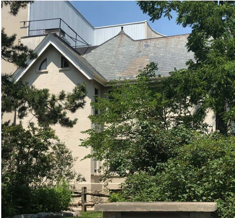
Figure 6 Current photograph looking north, showing the side (south) elevation of the Andrew Newton House at 10350 Yonge Street. Note the side gable with paneled bargeboard trim, quarter-round attic windows with rock-faced stone lugsills and brick voussoirs, and the metal ball finial surmounting the central hipped roof. (Source: HUD, 2023).
