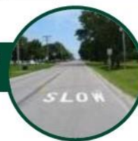
"SLOW" On-Road Sign Pavement Markings
