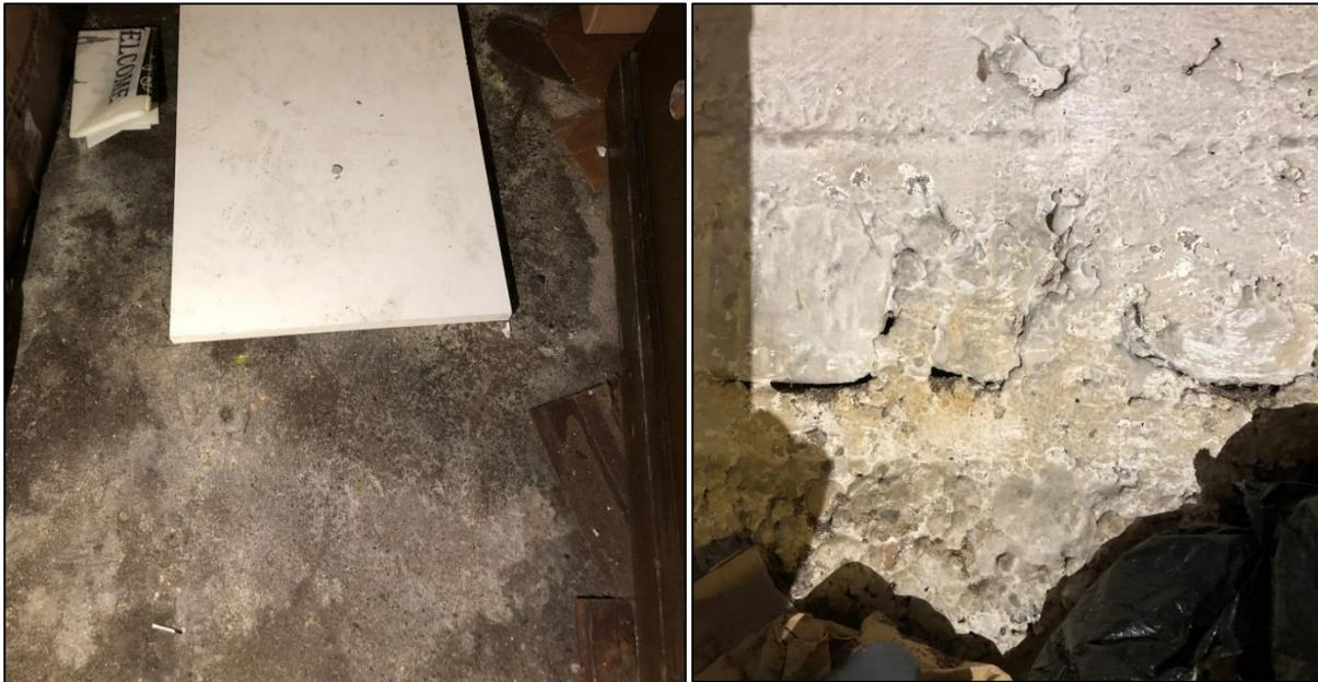
Figures 10, 11: Efflorescence and mold on the basement floor (left), and cracks in foundation wall (right).
