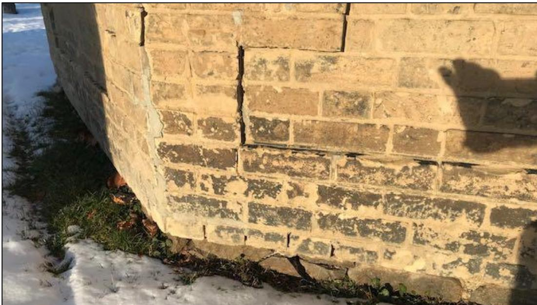
**Figure 17:** Typical damage to bricks on the exterior of the Octagonal Vault.
