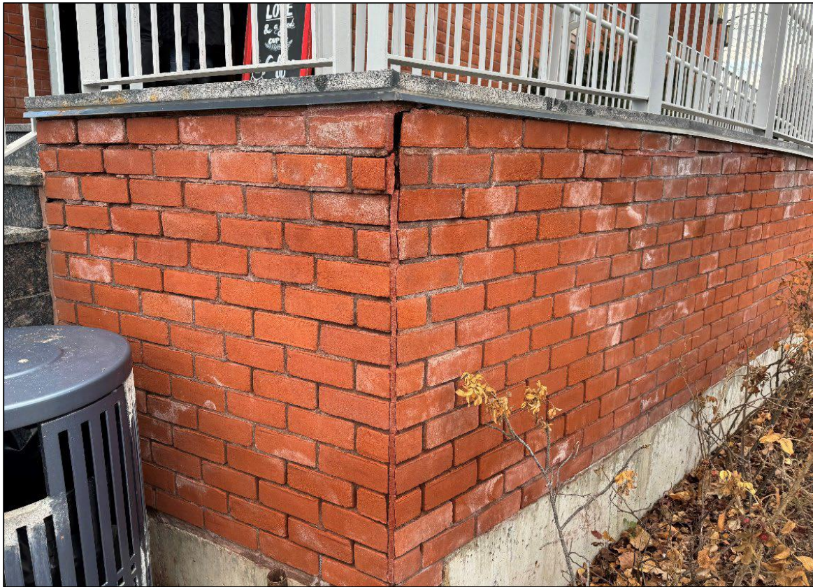
Figure 10: Flaking, failing mortar and efflorescence on ramp.
