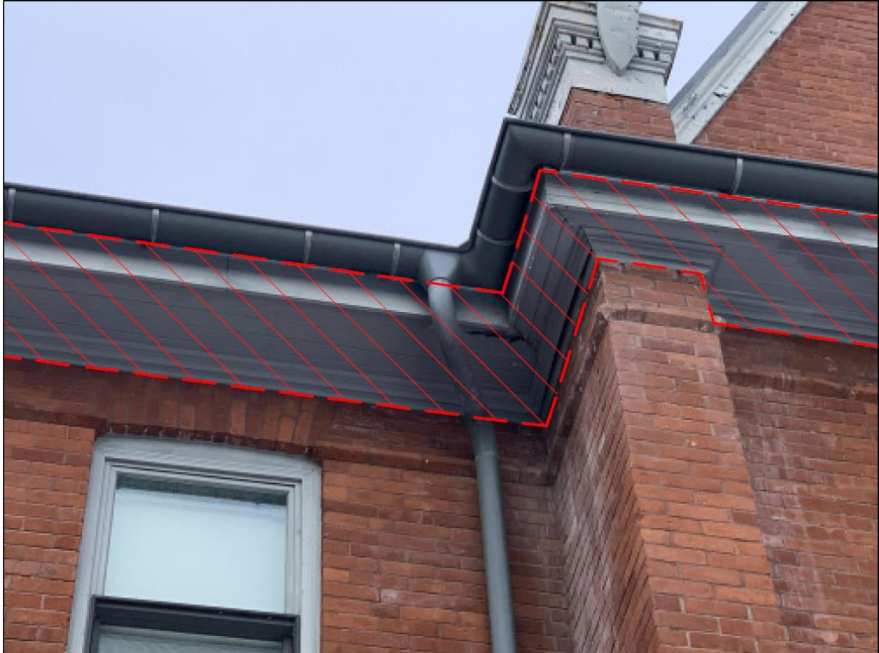
Figure 14: Damaged soffit board at corner, areas of peeling paint.
