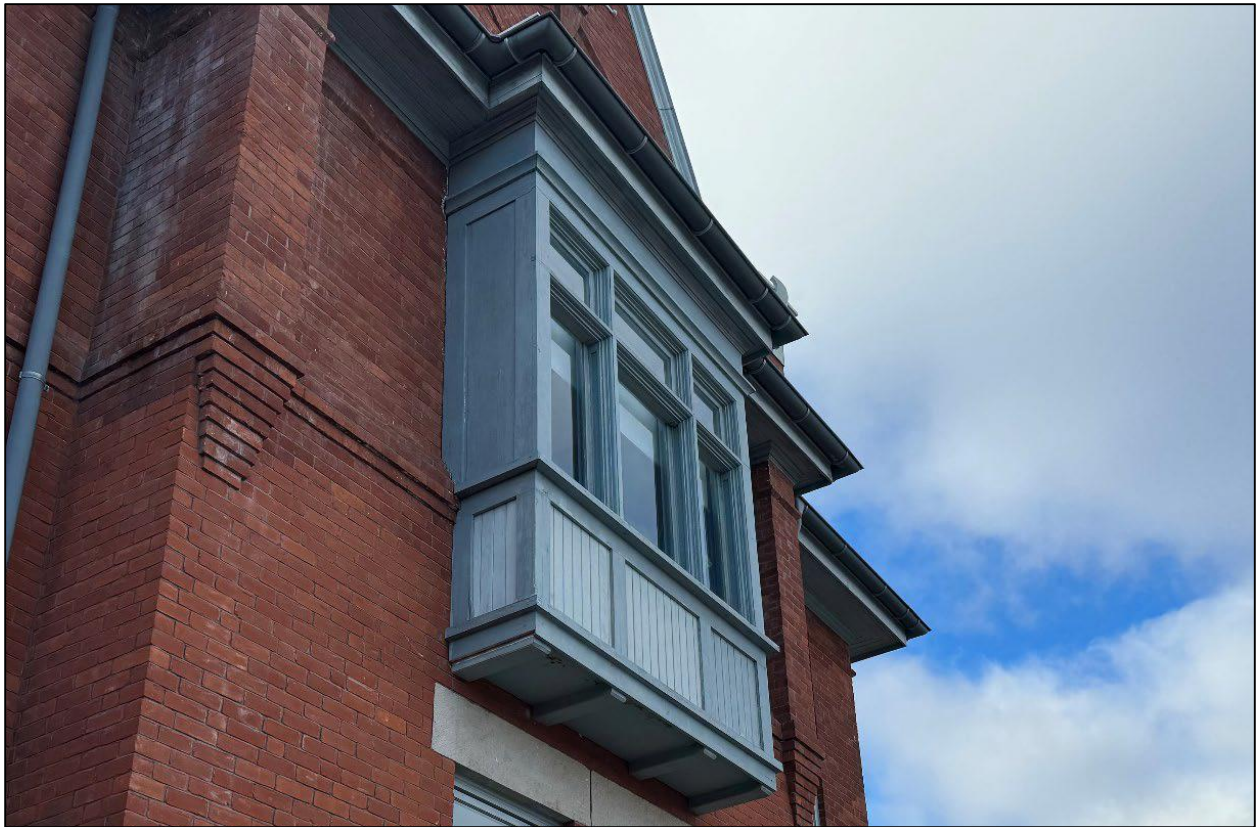
Figure 5: Paint peeling on the oriel window.
