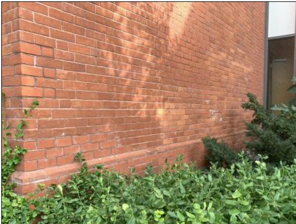
Figure 13: Areas of repointing done in with a mortar that does not match the original mortar colour.
