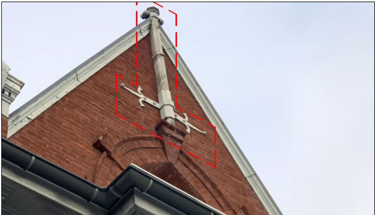
Figure 4: Peeling paint on gable roof trim and flagstaff.
