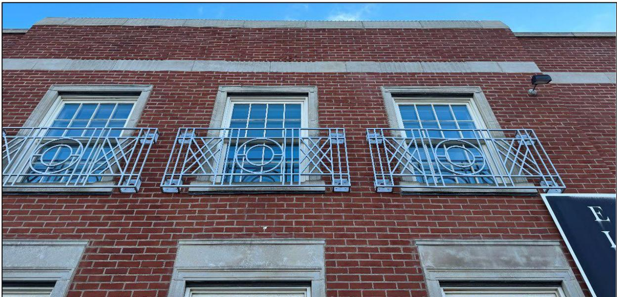
**Figure 2:** Decorative railing on upper storey windows on front façade.
