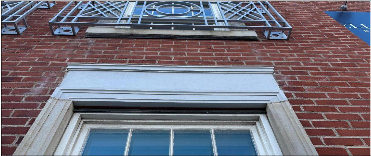
**Figures 8 and 9:** Examples of efflorescence on the front façade.
