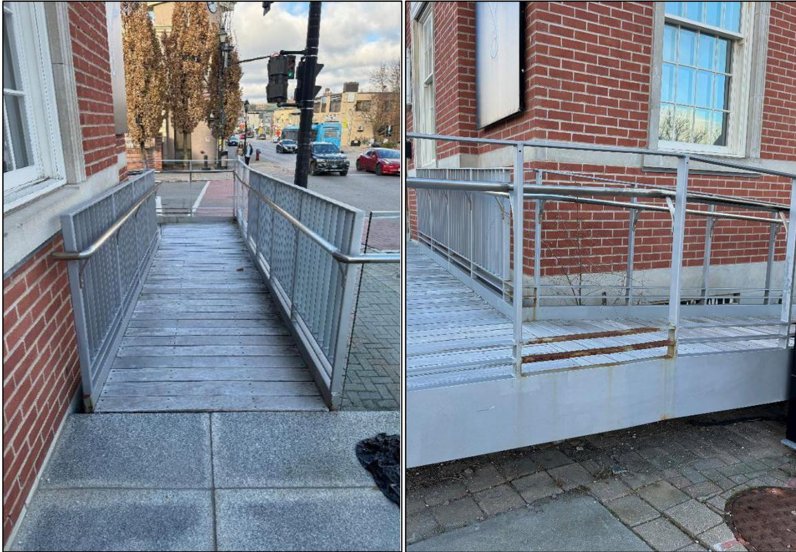
Figure 6 and 7: Planks showing areas of damage (left), rusted metal railings (right).
