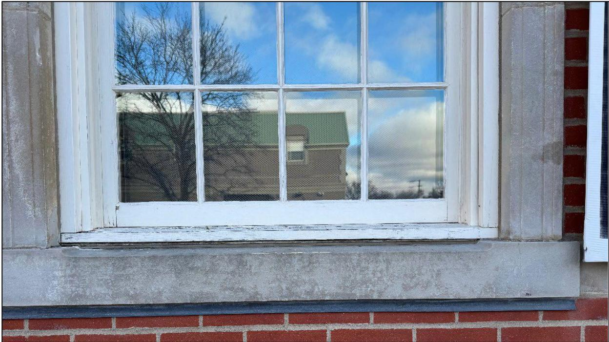
**Figure 5:** Window showing cracks, degraded paint.
