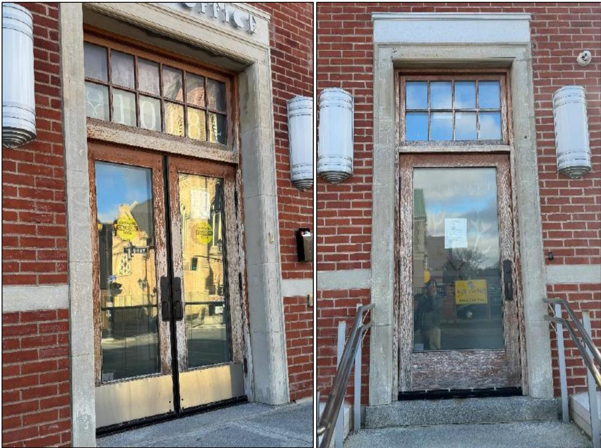
Figures 3 and 4: Front doors (left) and side door (right) exhibiting signs of deterioration.
