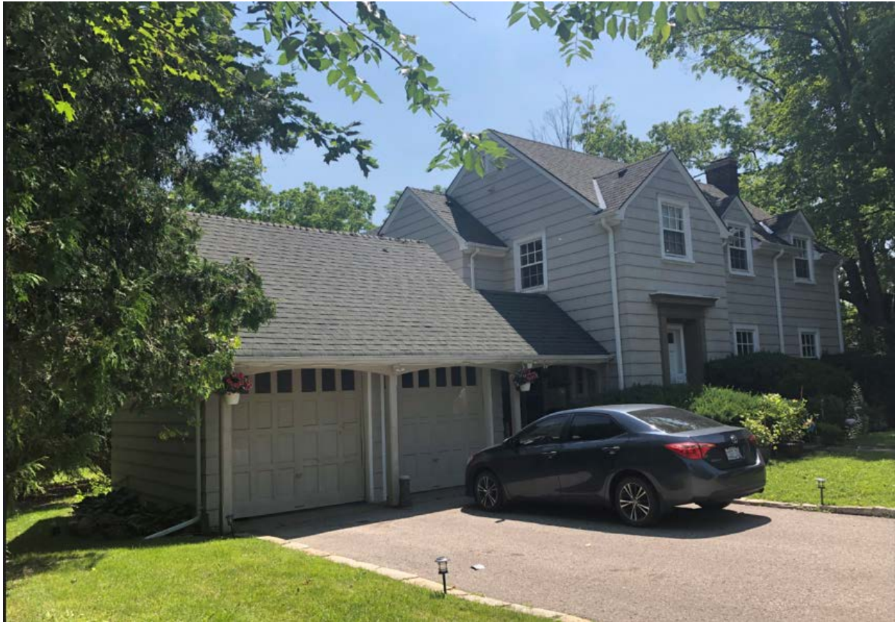
Figure 8 Photograph of the front (west) and side (north) elevations of the subject property at 27 Church Street North. Note the house's rectangular plan with attached garage, side-gabled roof with dormers, wide shingle cladding arranged in horizontal rows, the asymmetrical yet balanced composition of the front façade, the off-centre doorway with classical doorcase, and six-over-six window units (Source: HUD, 2023).
