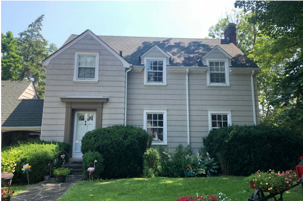
Figure 7 Photograph of the front (west) elevation of the subject property at 27 Church Street North. Note the house's rectangular plan with attached garage, side-gabled roof with dormers, wide shingle cladding arranged in horizontal rows, the asymmetrical yet balanced composition of the front façade, the off-centre doorway with classical doorcase, and six-over-six window units (Source: HUD, 2023).
