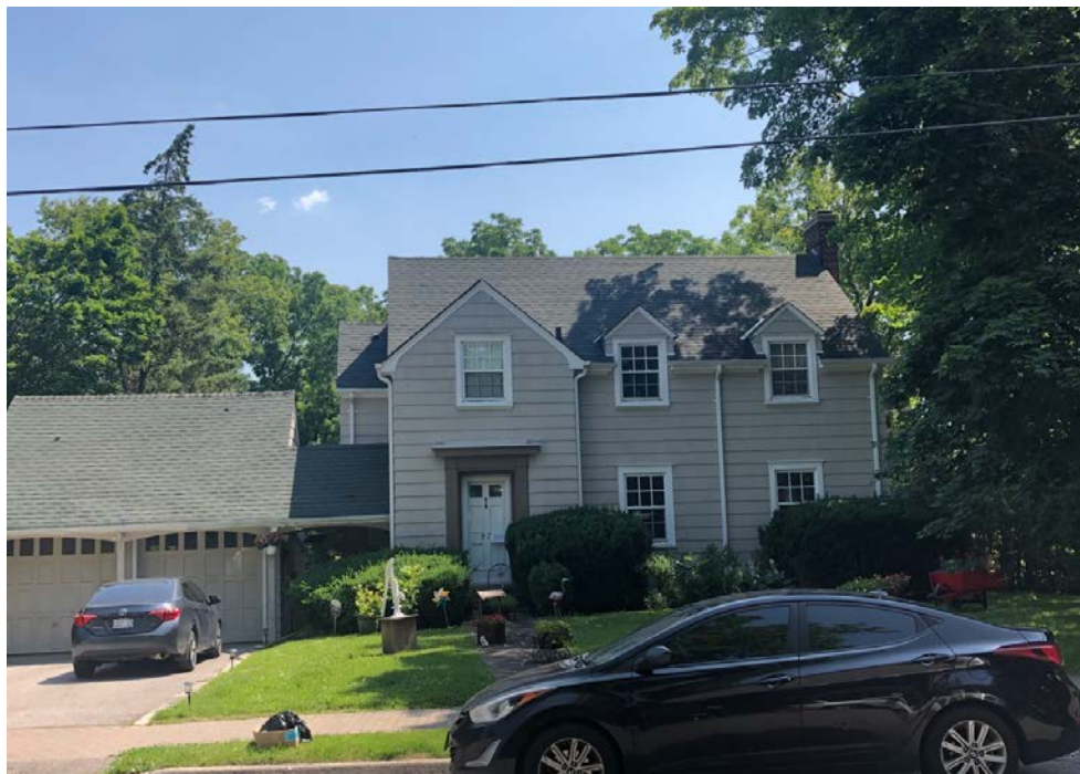
Figure 6 Photograph of the front (west) elevation of the subject property at 27 Church Street North. Note the house's rectangular plan with attached garage, side-gabled roof with dormers, wide shingle cladding arranged in horizontal rows, the asymmetrical yet balanced composition of the front façade, the off-centre doorway with classical doorcase, and six-over-six window units (Source: HUD, 2023).
