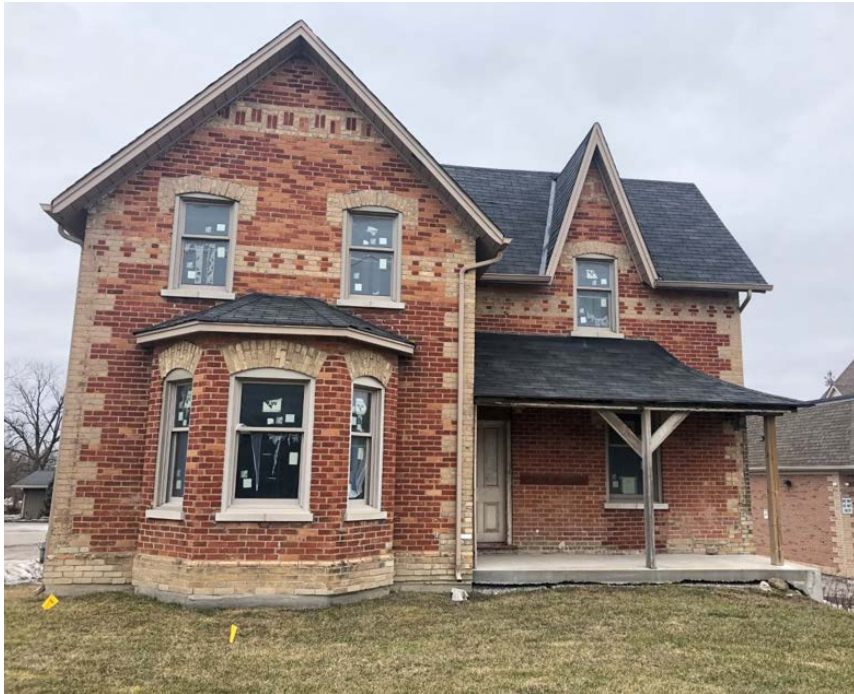
Figure 5 Photograph of the William Munro House's front (west) elevation, looking east from Leslie Street. Note the building's 1 ½-storey massing, medium-pitched cross-gabled roof with steep central gable on the building's ell, playful dichromatic brickwork, segmental arched windows, projecting bay window with hipped roof, and main entrance with a paneled wooden door and bellcast-roofed verandah (Source: HUD, 2024).
