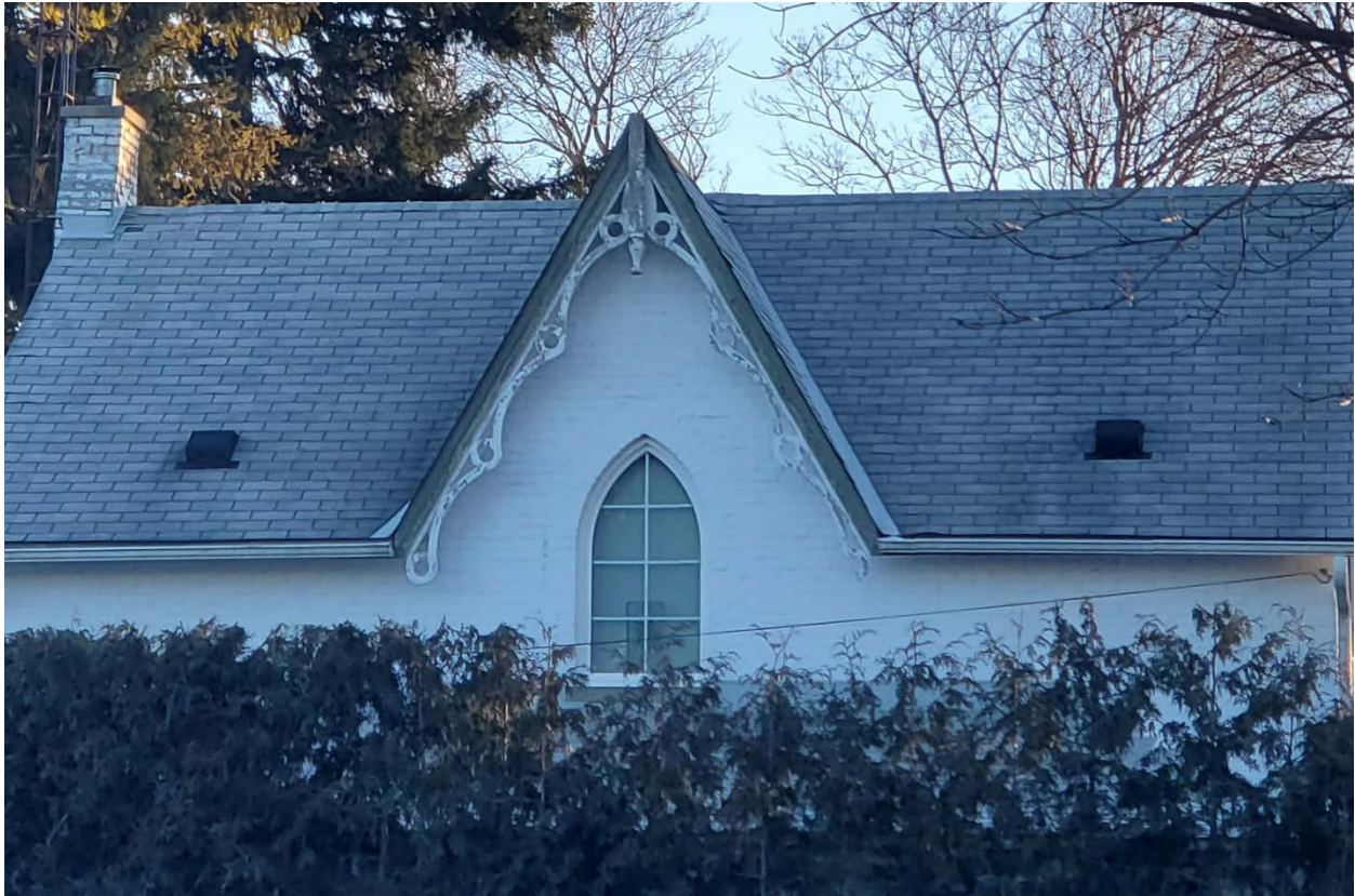
Figure 6 Current photograph looking east, showing the principal (west) elevation of 13561 Leslie Street. Note the structure's vergeboarding, finial, and lancet arch window. (Source: HUD 2024)
