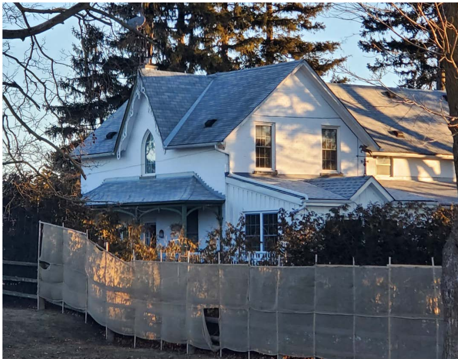
Figure 5 Current photograph of the Forester House looking northeast, showing the principal (west) and south elevations. Note the building's 1 ½ storey massing, side gable roof with front gable, and wooden porch with bellcast roof. (Source: HUD 2024)
