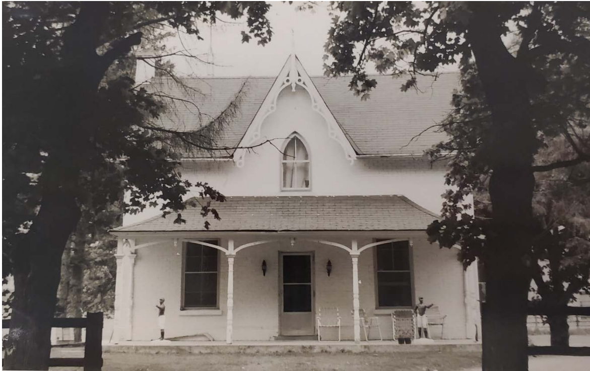
Figure 4 1984 photograph of the Forester House, taken from Leslie Street looking east. Note the structure's symmetrical front façade, lancet arch window, vergeboarding, finial, and porch with bellcast roof and elliptical drops. (Source: Richmond Hill Local Architectural Conservation Advisory Committee)
