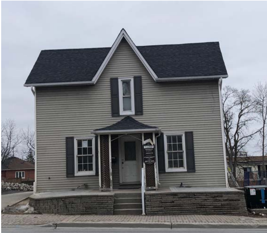
Figure 6 Photograph of 10039 Yonge Street's front (west) elevation, looking east from Yonge Street. Note the building's 1 ½-storey massing, simple, rectangular plan, medium-pitched side-gabled roof, central dormer inset with a narrow second-storey window, the balanced composition of its front (west) façade, flat-headed window and door openings, and central portico entry (Source: HUD, 2024).
