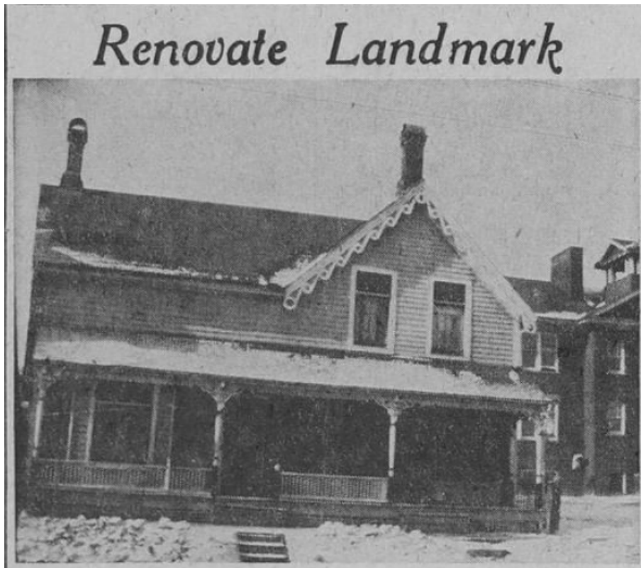
Figure 7 1955 photograph of the Jerry Smith Building at 10094 and 10096 Yonge Street published in the Liberal . Note the building's distinctive "scroll" bargeboard trim and full-façade verandah with turned wooden posts and decorative brackets. (Source: Liberal , Apr 15, 1955)
