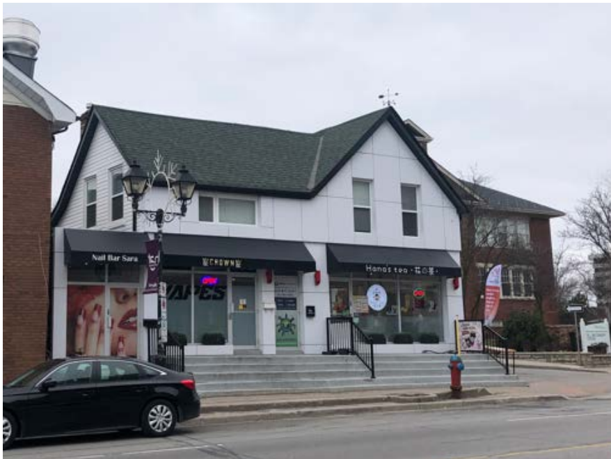
Figure 11 Photograph of the Jerry Smith Building's front (east) and partial south (side) elevations, looking northwest from Yonge Street. Note the building's 1 ½-storey massing, medium-pitched cross-gabled roof with front (east) and south gable ends, flat headed windows, and storefronts at grade. (Source: HUD, 2024)
