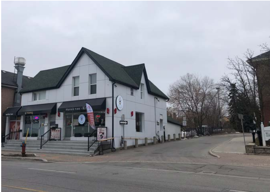
Figure 10 Photograph of the Jerry Smith Building's front (east) and side (north) elevations, looking southwest from Yonge Street. Note the building's 1 ½-storey massing, L-shaped plan, medium-pitched cross-gabled roof with front (east) gable end and north gable, flat headed windows, and storefronts at grade. (Source: HUD, 2024)
