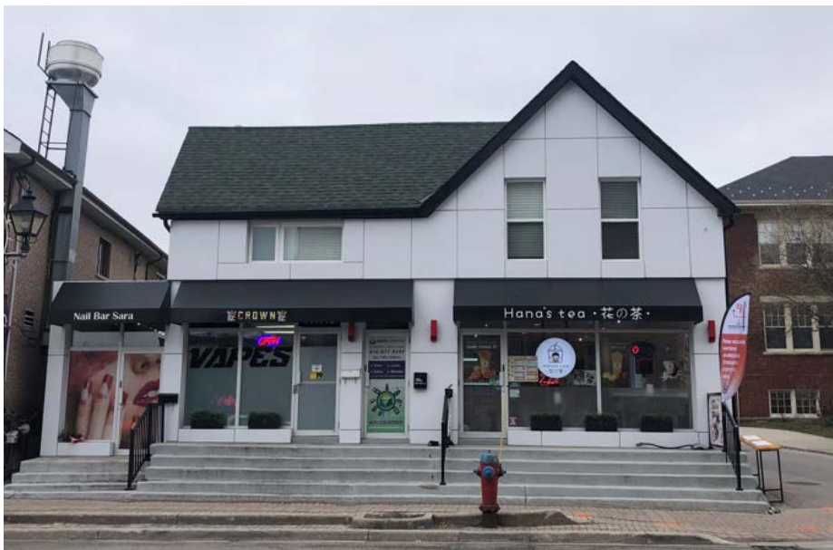
Figure 9 Photograph of the Jerry Smith Building's front (east) elevation, looking west from Yonge Street. Note the building's 1 ½-storey massing, medium-pitched cross-gabled roof with front (east) gable end, flat headed windows, and storefronts at grade. (Source: HUD, 2024)
