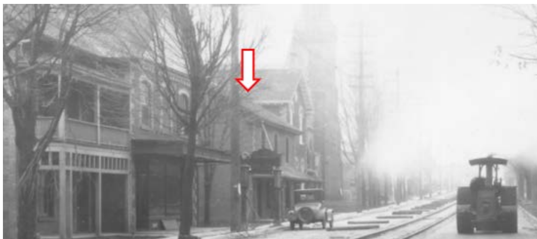
Figure 3 C1927 photograph of the John Coulter Tailor Shop (indicated by the arrow), taken from Yonge Street looking southeast. Photograph indicates that the building was originally red brick with buff brick quoins on the front (west) façade. (Source: Richmond Hill Public Library Digital Archive)
