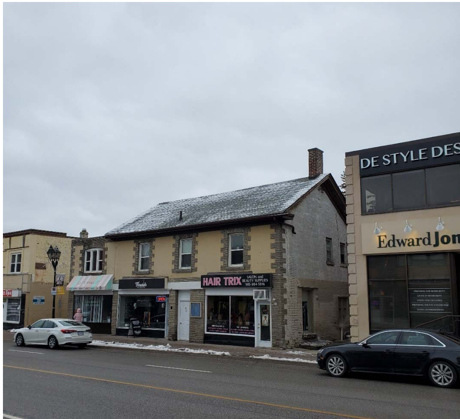
Figure 7 Current photograph of 10217 Yonge Street looking northeast, showing the site's context on Yonge Street. Note the surrounding small-scale commercial structures. (Source: HUD, 2024)
