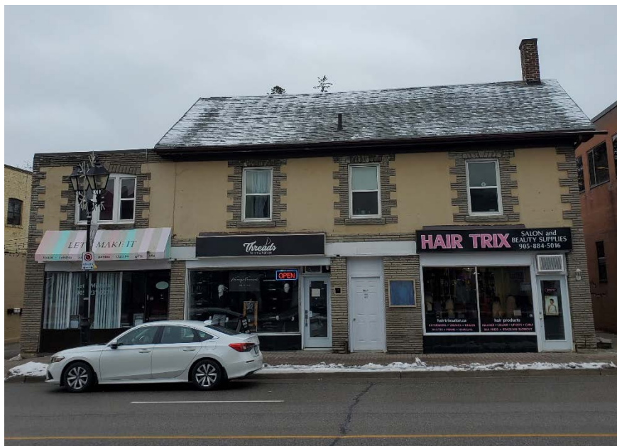
Figure 5 Current photograph looking east, showing the principal (west) elevation of 10217 Yonge Street. Note the building's two-storey massing, side gable roof, and symmetrical three-bay front (west) façade on the main portion of the building. (Source: HUD, 2024)
