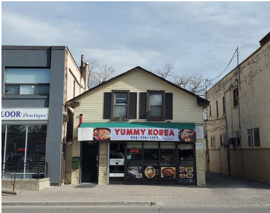
Figure 5 Current photograph looking east, showing the principal (west) elevation of 10231 Yonge Street. Note the building's 1 ½ storey massing, front-gable roof with return eaves, and frame construction. (Source: HUD, 2024)
