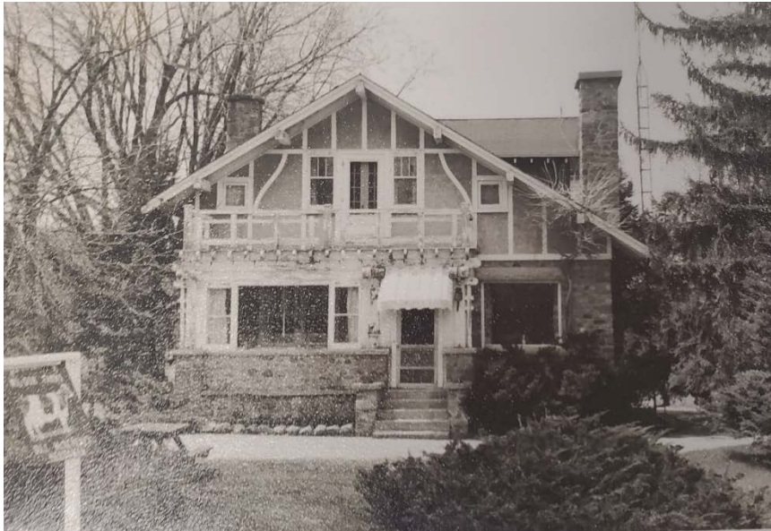
Figure 4 Circa 1980s photograph of the Mitchell-Durham House at 12800 Yonge Street. Note the asymmetrical but balanced front façade, cobblestone and stucco exterior, front gable roof, enclosed front porch, cobblestone chimneys, and decorative half-timbering. (Source: Richmond Hill Local Architectural Conservation Authority Committee)
