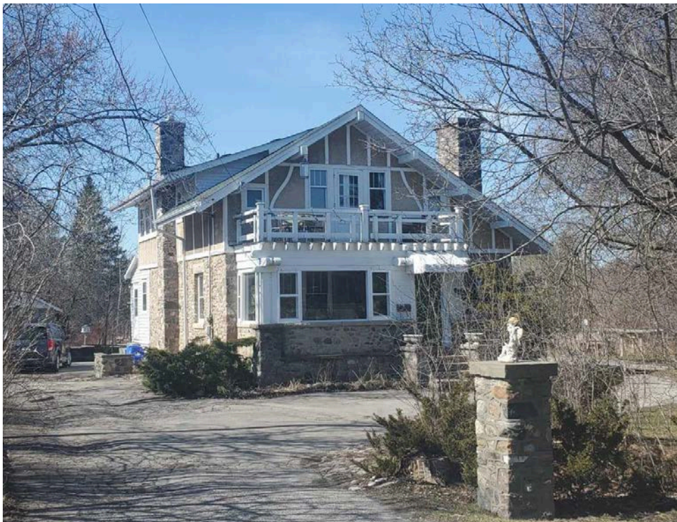
Figure 5 Current photograph of the Mitchell-Durham House at 12800 Yonge Street showing the front (east) elevation. Note the 1 ½ storey massing, asymmetrical but balanced front façade, cobblestone and stucco exterior, front gable roof, enclosed front porch, cobblestone chimneys, and decorative half-timbering. (Source: HUD, 2024)
