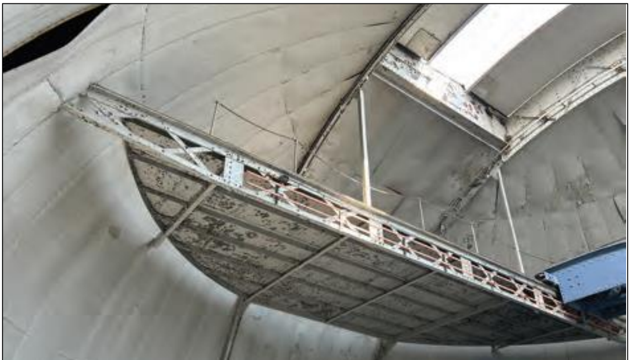
Figure 5 The upper portion of the dome showing degraded Agasote panels and peeling paint (Source: +VG Architects).
