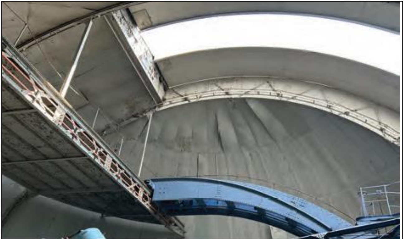
Figure 4 The upper portion of the dome showing degraded Agasote panels and peeling paint (Source: +VG Architects)
