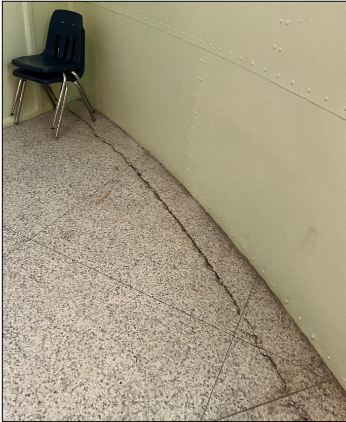
Figure 6 A portion of the crack in the terrazzo flooring that runs parallel to the exterior Observatory wall (Source: City of Richmond Hill).
