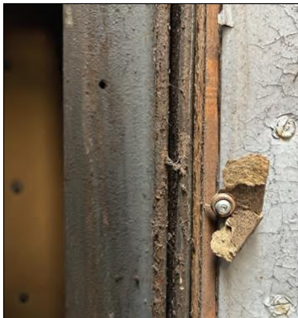
Figures 10, 11 Panel removed to show underlying wood strapping and supporting metal structure (left); illustration of how existing panels overlap and are attached to the steel girder (Source: +VG Architects).
