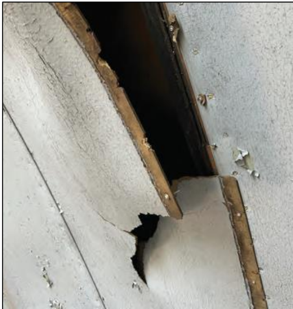
Figures 1-3 Agasote panels showing degradation, including warping, peeling, and failed joints (Source: +VG Architects)
