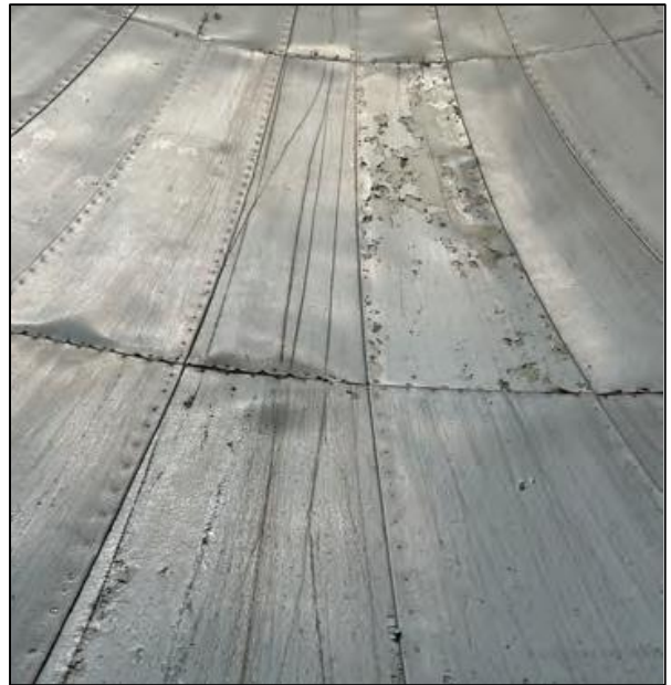
Figures 1-3 Agasote panels showing degradation, including warping, peeling, and failed joints (Source: +VG Architects)
