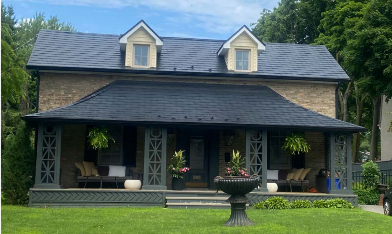
Figure 1 July 2024 photograph of 165 Richmond Street's main (south) elevation, showing the replica bellcast-roofed front verandah on decorative treillage supports (Source: HUD 2024).
