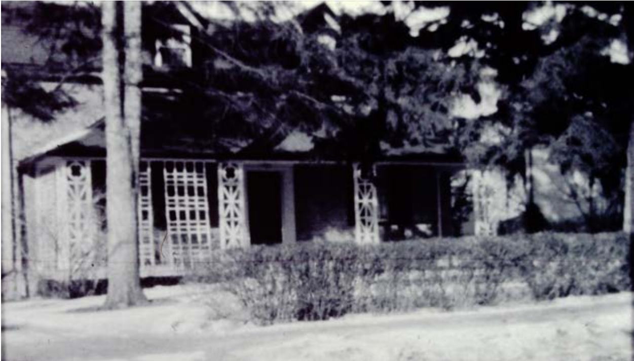
Figure 2 C. 1980s archival photograph of 165 Richmond Street's main (south) elevation, showing the historical bellcast-roofed front verandah on decorative treillage supports (Source: Richmond Hill Public Library Local History and Genealogy Collection).
