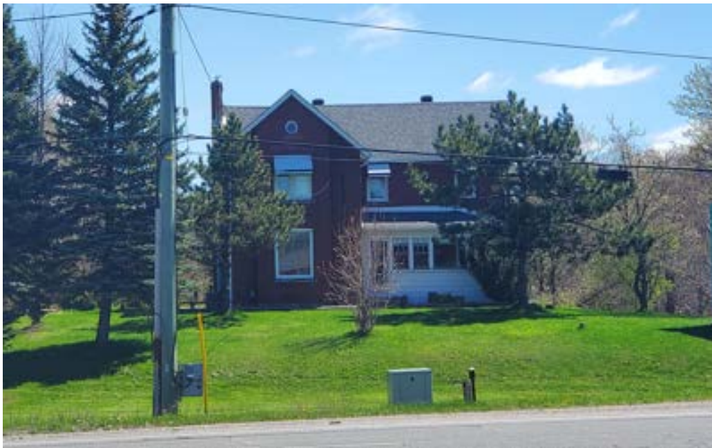
Figure 3 Current photograph of the Ryan-Paxton House at 12345 Yonge Street, showing the building's principal (west) elevation. Note the building's 2-storey massing, red brick veneer, complex cross-gabled roof, projecting bay, enclosed hipped-roof front verandah, and roundel attic window. (Source: HUD, 2024)
