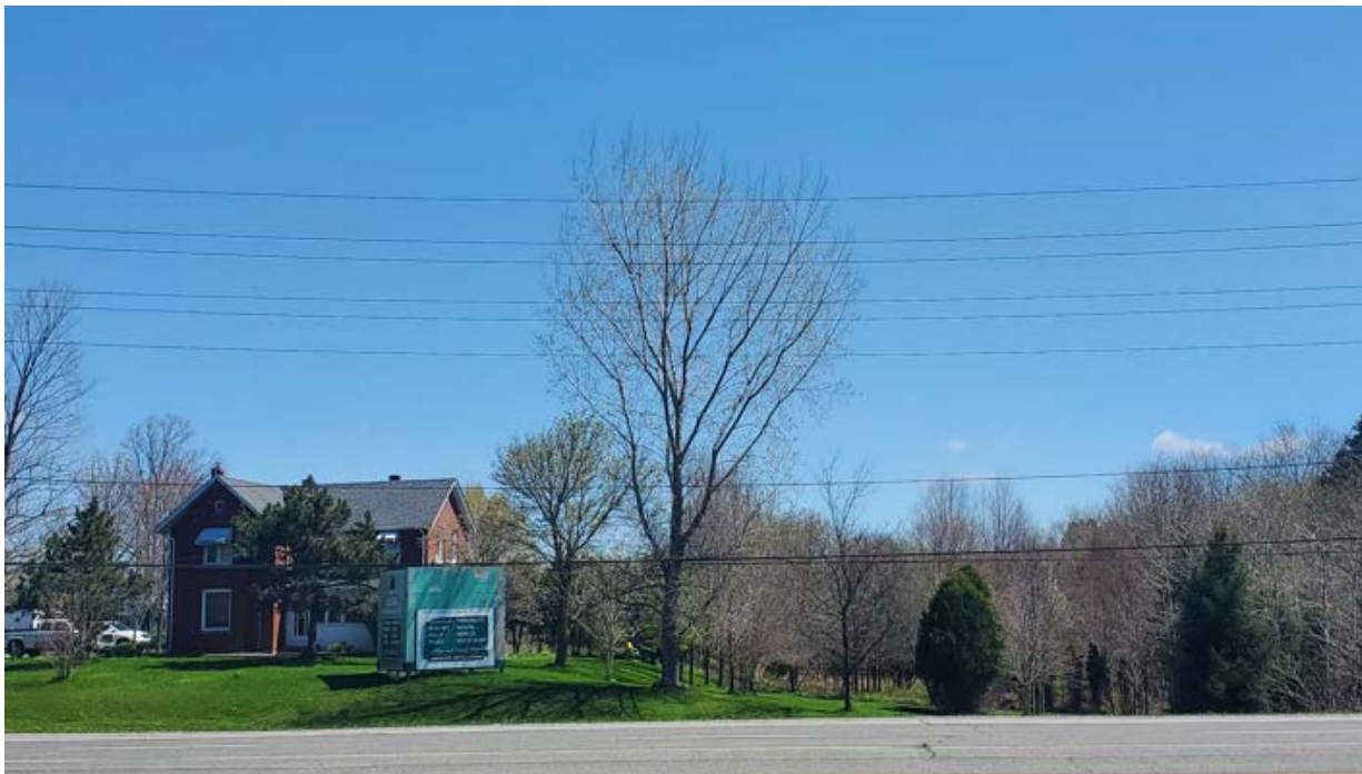
Figure 5 Current photograph of the Ryan-Paxton House at 12345 Yonge Street facing east. Note the surrounding context, including the sparse development and thick vegetation. (Source: HUD, 2024)
